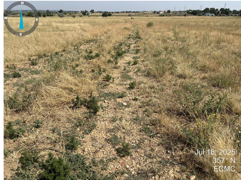
Photo 2. Picture taken on the south end of the access road looking north. Gravel remains on the southern part of the access road. Vegetation establishment is lower on the former access road than surrounding area.
