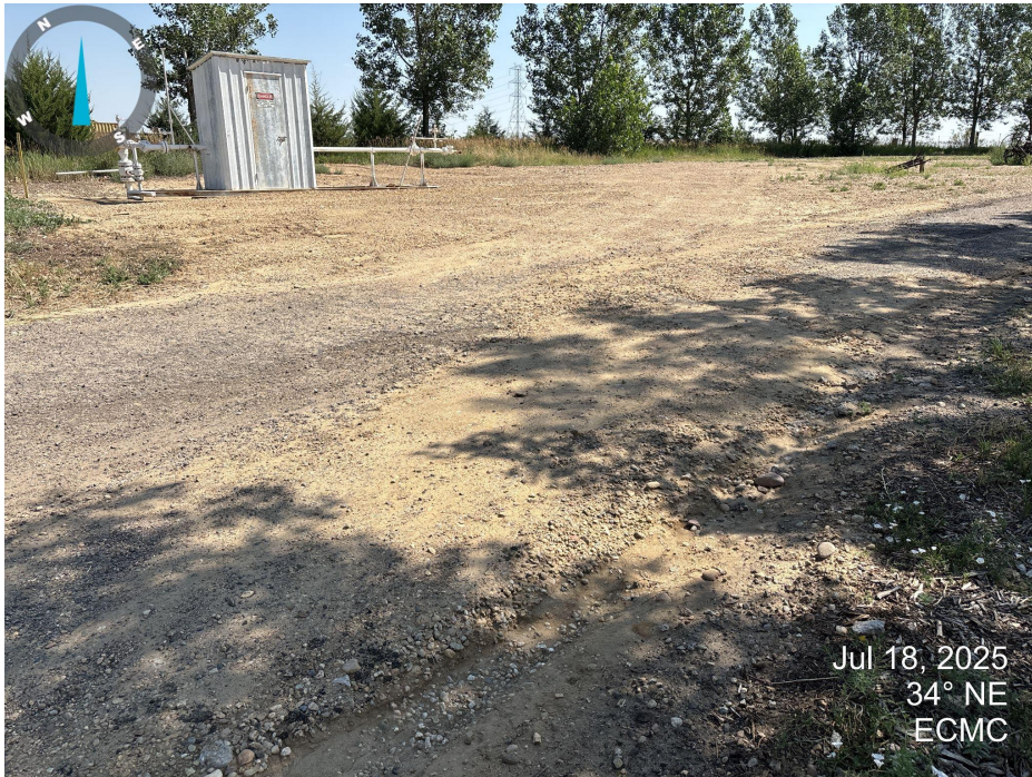
Photo 5. Looking north across the west side of location. Sediment and gravel washing over the road.
