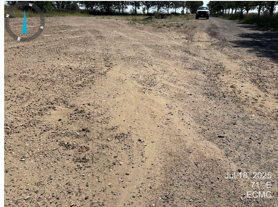
Photo 4. Picture taken on the east side of the location. Stormwater erosion channels are beginning to form on location and sediment is leaving the site.
