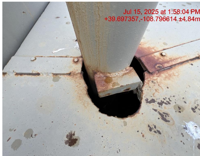
Photo # 9998 Hole in separator building open to wildlife/available for entry by wildlife
