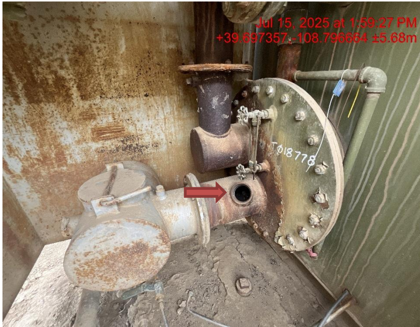
Photo # 9999 Separator heater open to wildlife/available for entry by wildlife
