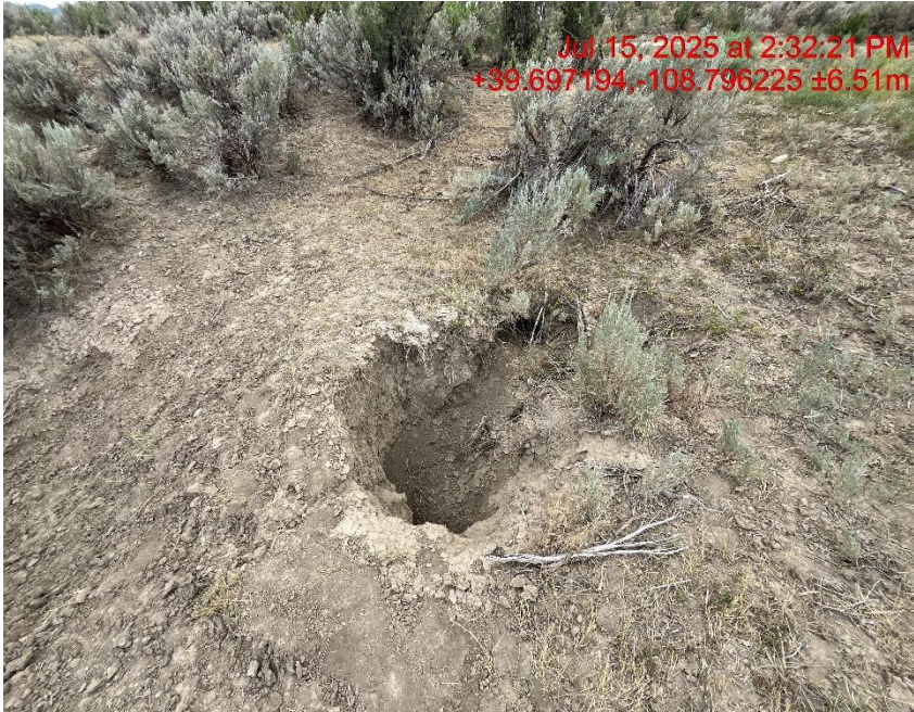
Photo # 0028 Subsidence on SE side of location, additionally is a wildlife hazard/personnel safety hazard
