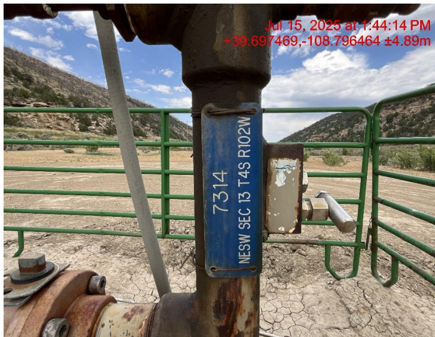
Photo # 9986 Wellhead sign lacks required information/not in compliance with CECMC rules
