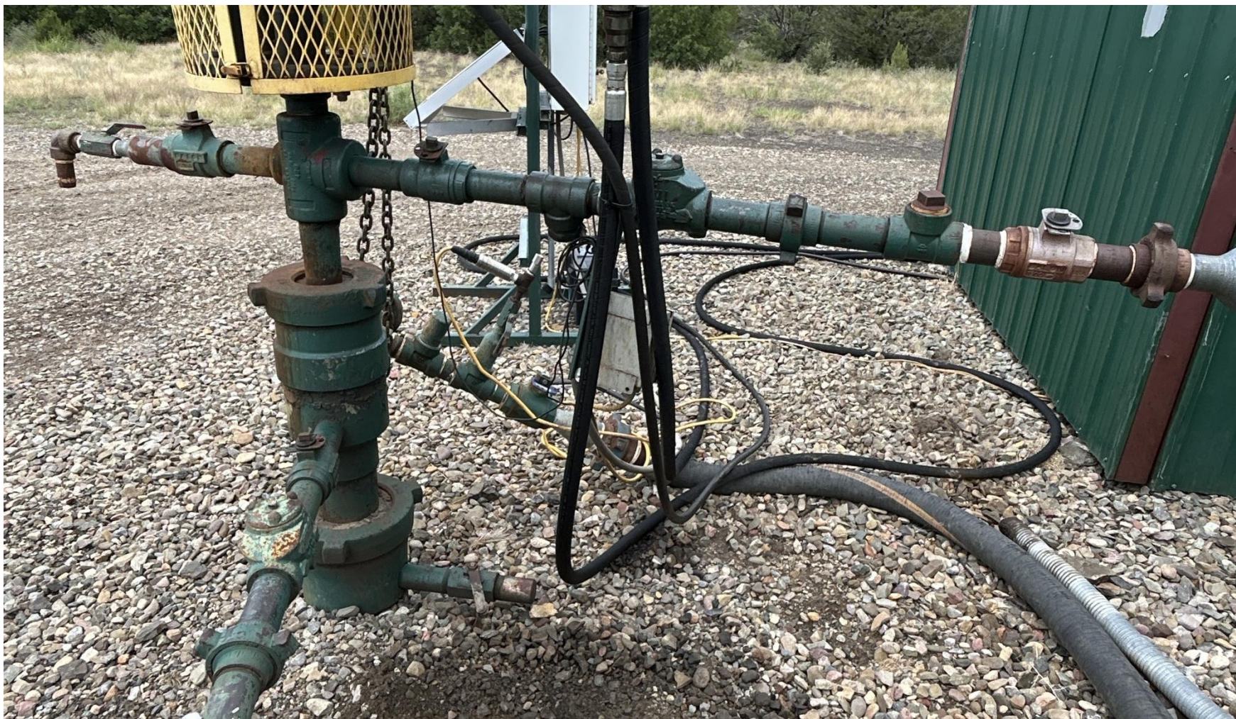
PHOTO 3: WELLHEAD & STAINED SOIL
