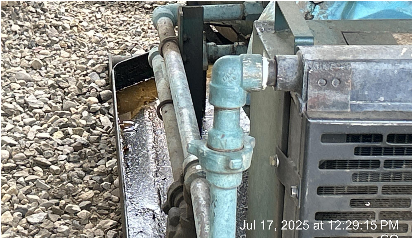
PHOTO 4: OIL IN LIQUID RING SKID
