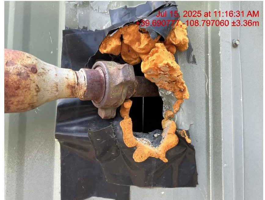
Photo # 9896 Hole in meter house open to wildlife/available for entry by wildlife
