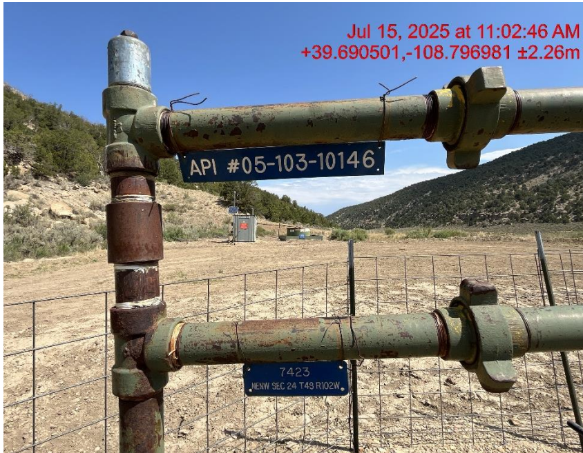
Photo # 9883 Wellhead sign lacks required information/not in compliance with CECMC rules
