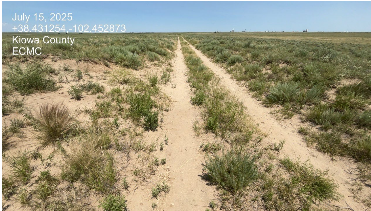
Photo 2. Facing north along the access road. The road needs to be recontoured to original grade and reclaimed.
