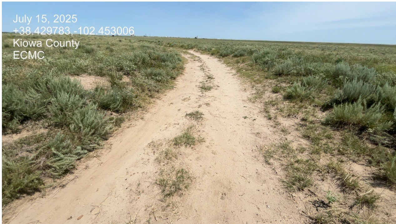
Photo 1. Facing northeast along the access road. The road needs to be recontoured to original grade and reclaimed.
