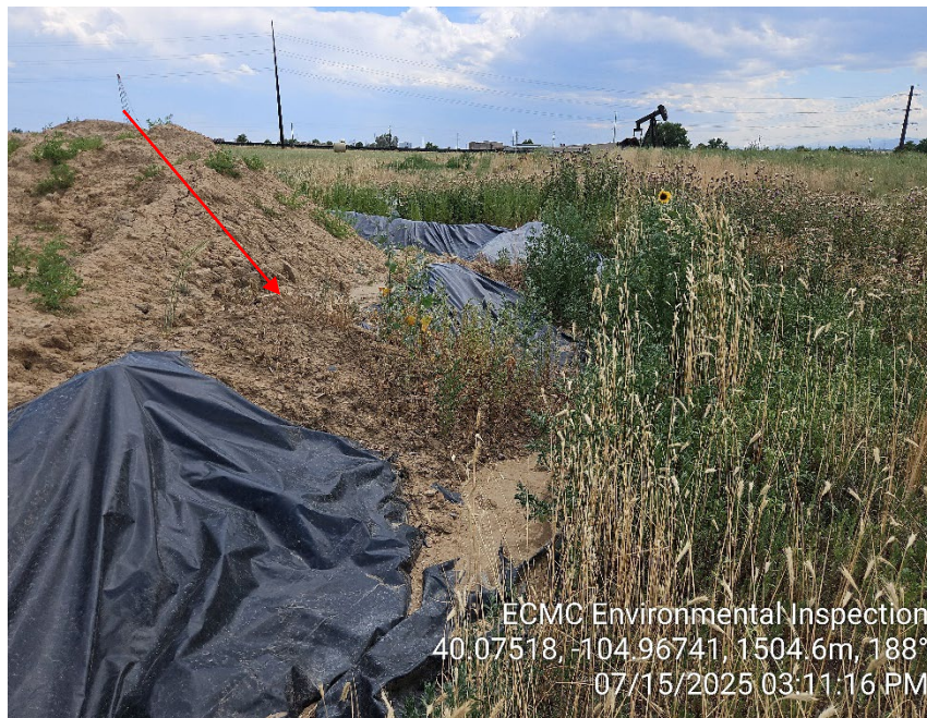
Photo 21 – Contaminated stockpile. Inadequate BMPs; observed sediment transport. Weeds.
