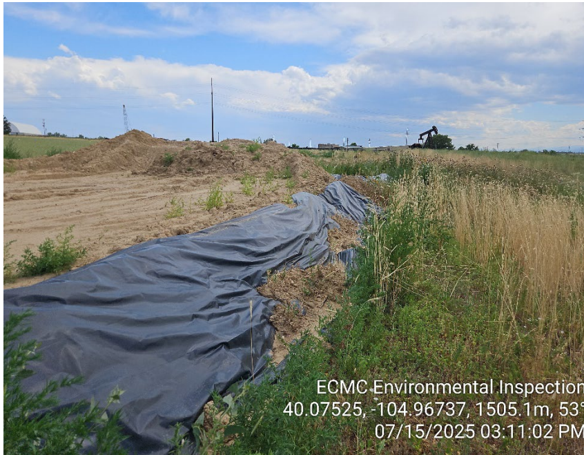
Photo 19 – Contaminated stockpile. Inadequate BMPs. Weeds.
