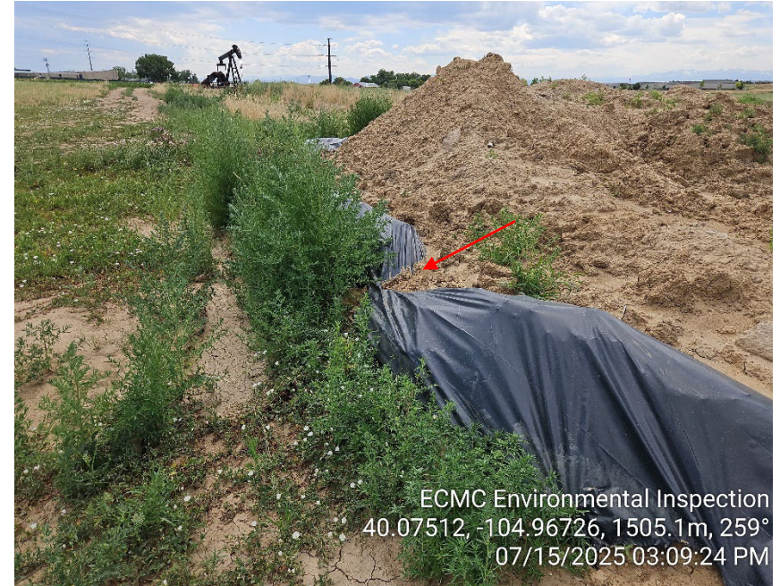
Photo 14 - Contaminated stockpile. Inadequate BMPs; observed sediment transport. Weeds.
