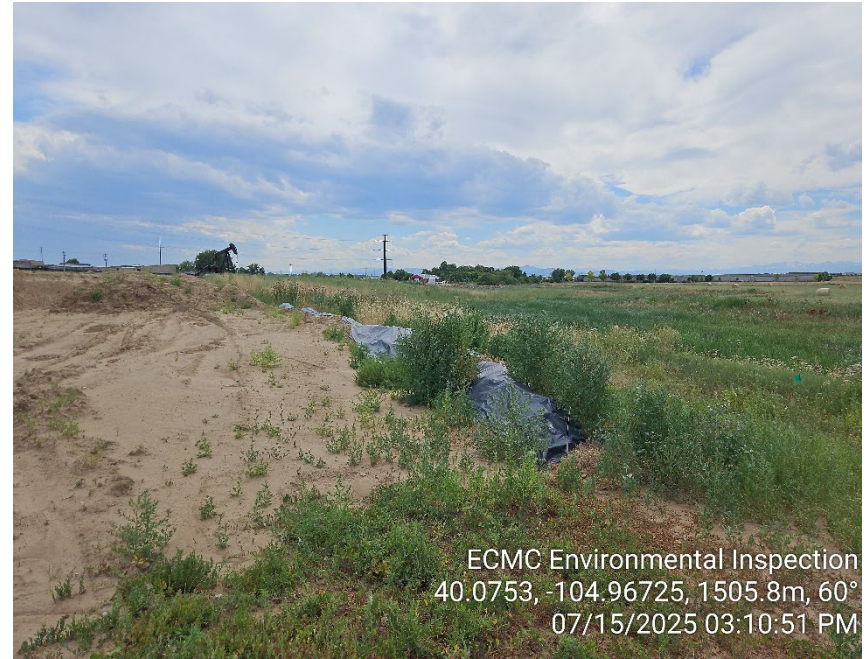
Photo 20 - Contaminated stockpile. Inadequate BMPs. Weeds.
