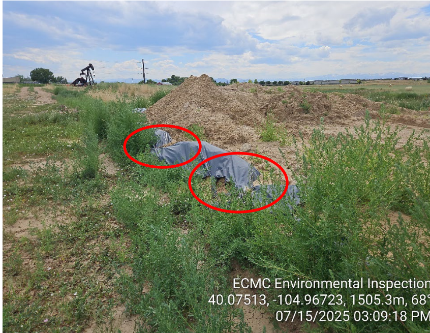
Photo 13 – Contaminated stockpile. Inadequate BMPs with torn liner and observed sediment transport. Weeds.
