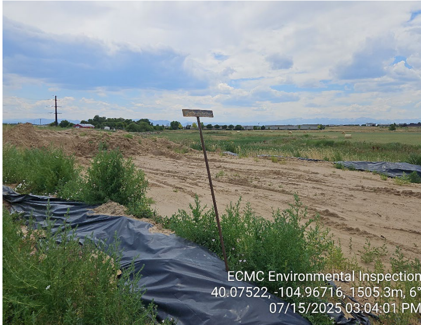
Photo 11 – Contaminated stockpile. Inadequate BMPs. Weeds.
