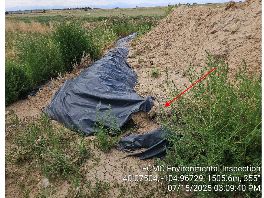
Photo 16 - Contaminated stockpile. Inadequate BMPs; observed sediment transport & torn liner. Weeds.
