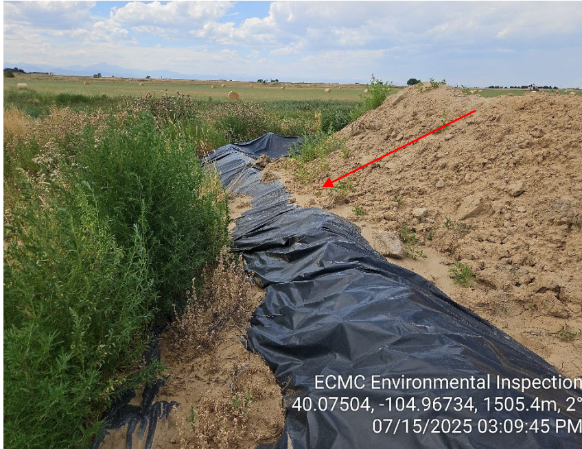
Photo 17 – Contaminated stockpile. Inadequate BMPs; observed sediment transport. Weeds.
