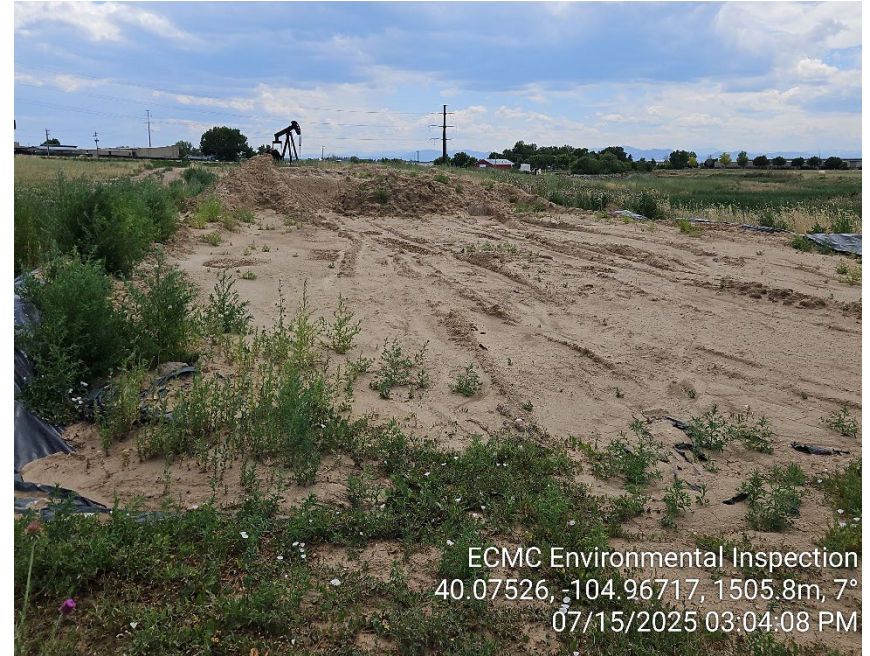
Photo 12 - Contaminated stockpile. Inadequate BMPs. Weeds.
