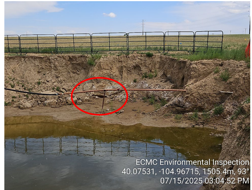
Photo 8 - Open excavation. Hydrocarbon impacts visible on south excavation sidewall. Downed fencing/weeds.
