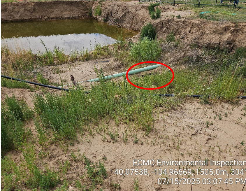
Photo 9 – Open excavation with weeds. Impacts visible below pipeline.
