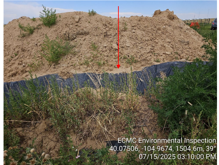
Photo 18 - Contaminated stockpile. Inadequate BMPs; observed sediment transport. Weeds.
