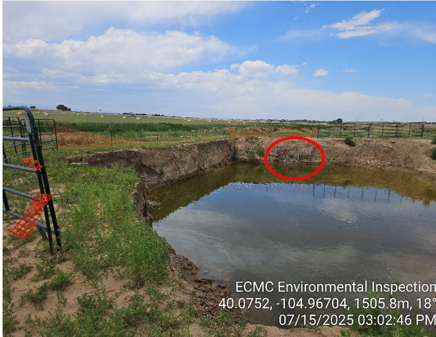
Photo 3 – Open excavation. Sheen observed on groundwater. Hydrocarbon impacts visible on north excavation sidewall. Downed fencing/weeds.
