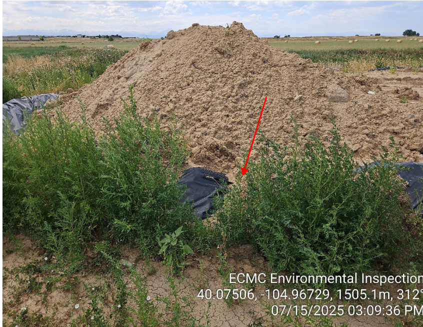
Photo 15 – Contaminated stockpile. Inadequate BMPs; observed sediment transport. Weeds.
