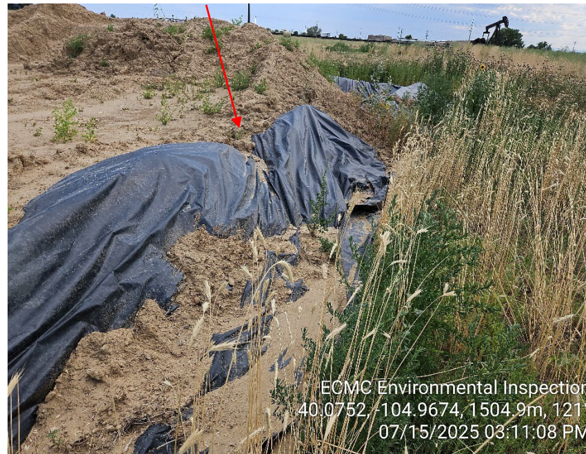
Photo 22 - Contaminated stockpile. Inadequate BMPs; observed sediment transport. Weeds.
