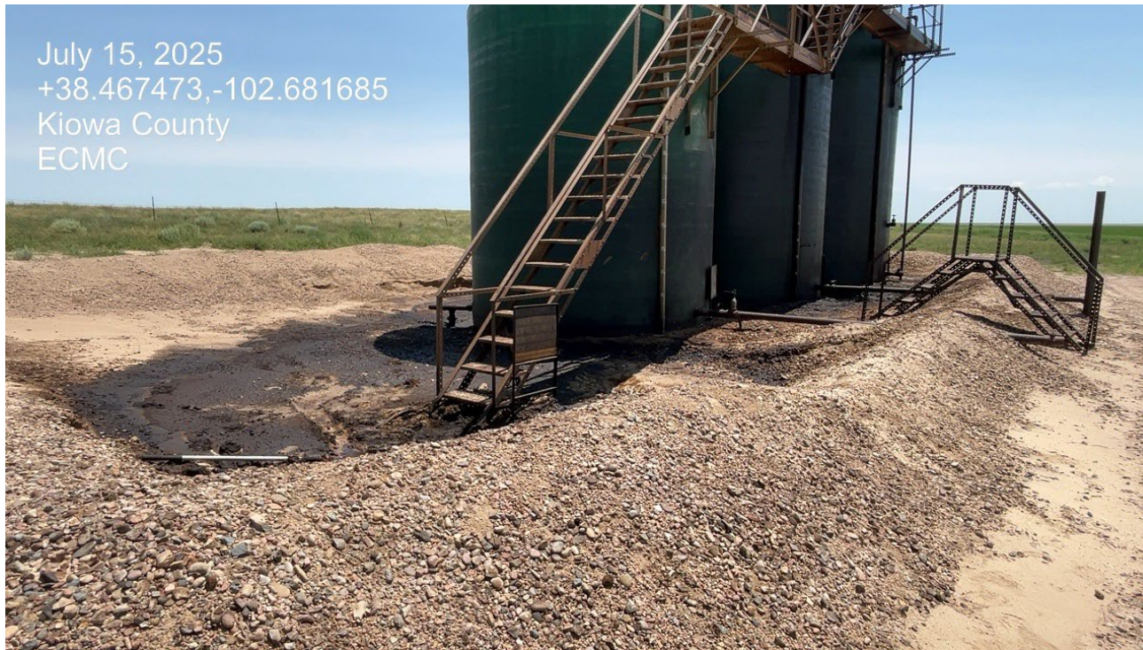
Photo 2. Facing toward the tank battery. There is a new recent spill that has occurred which will need to be reported and cleaned up.
