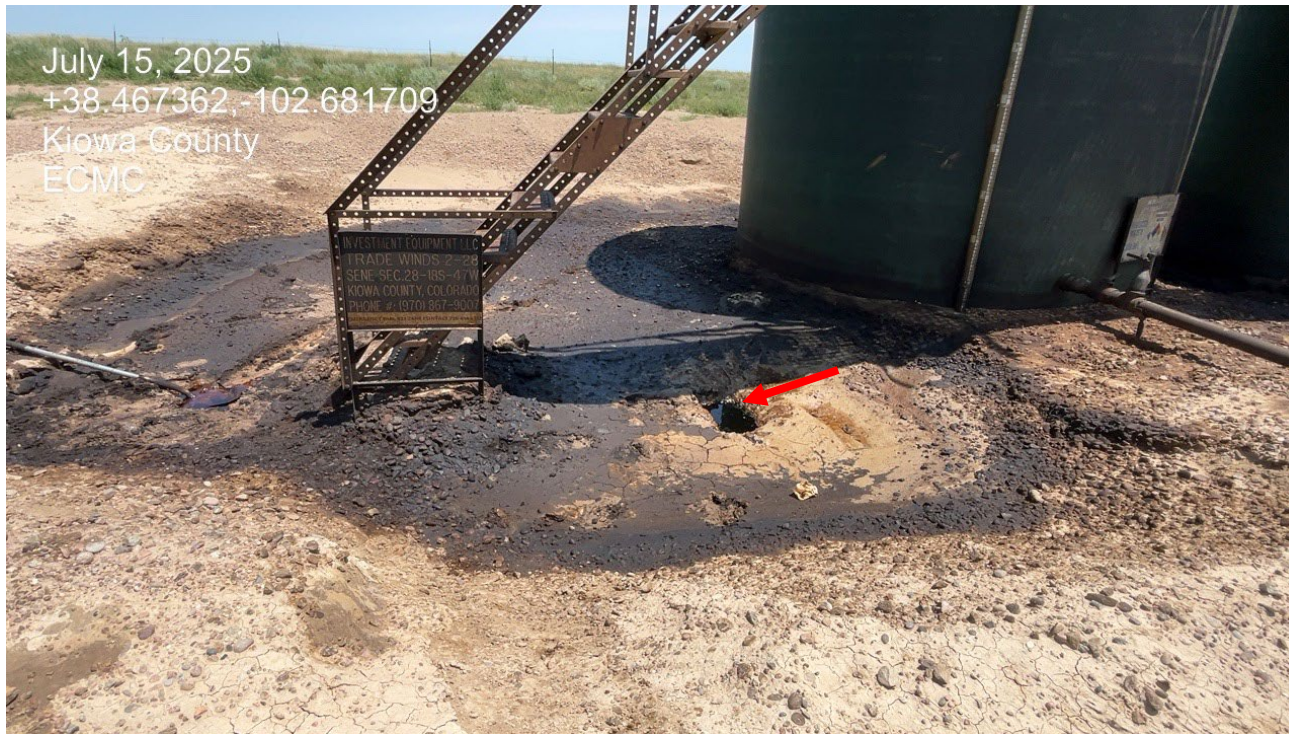
Photo 3. View of inside the containment shows signs of a recent spill with oily freestanding liquids shown at red arrow.
