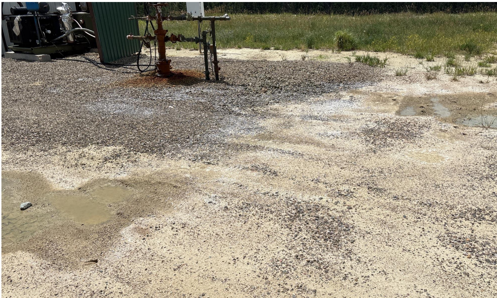
PHOTO 5: Produced water spill from the wellhead has left a salt and rust colored impacted area around the wellhead. Securely fasten all valves, pipes, fittings, and Production Facilities to ensure good mechanical condition, inspect at regular intervals and maintain in good mechanical condition remove and dispose of impacted material per Rule 608.e. CA DATE 7 .
