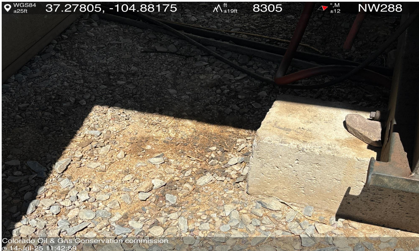
PHOTO 9: AREA OF IMPACTED SOIL PRIME MOVER ENGINE SKID. Conduct maintenance on equipment, cleanup stained material and review self inspection processes. COMPLY WITH RULE 1002,.(2).D. CA DATE 7-25-2025.
