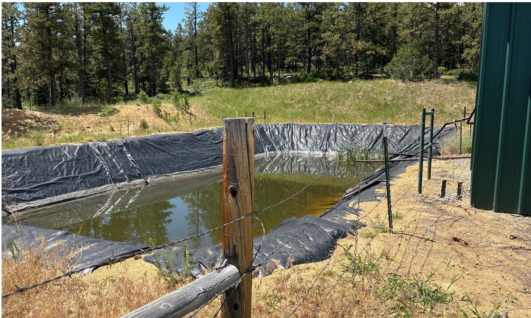
PHOTO 4: PRODUCED WATER PIT.
