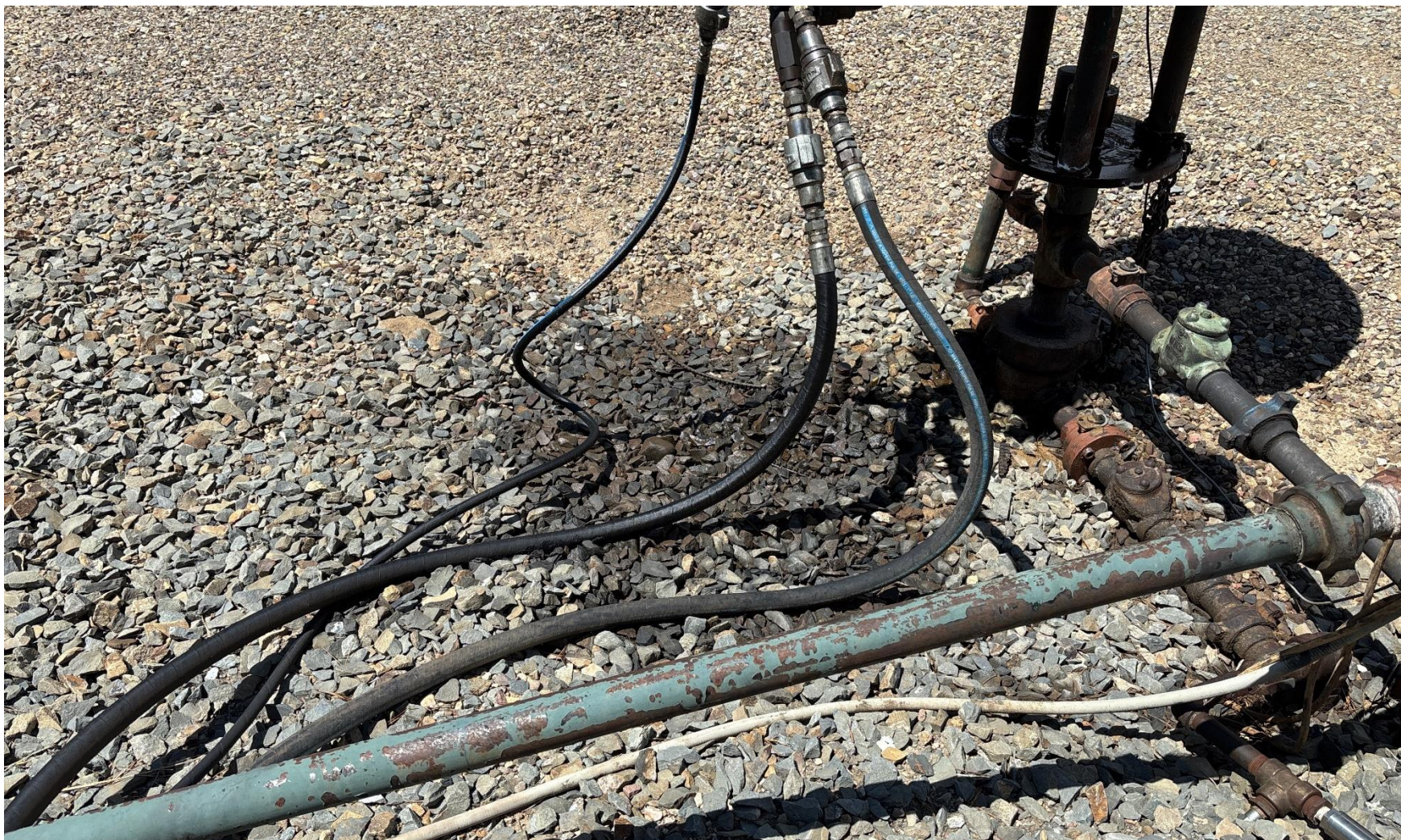
PHOTO 6: AREA OF IMPACTED SOIL NEAR WELLHEAD. Conduct maintenance on equipment, cleanup stained material and review self inspection processes. COMPLY WITH RULE 1002,.(2).D. CA DATE 7-25-2025.
