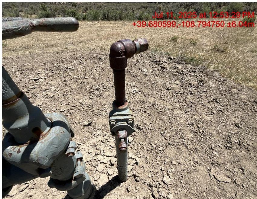
Photo # 9724 Unused flowline does not comply with CECMC 600 & 1100 series rules
