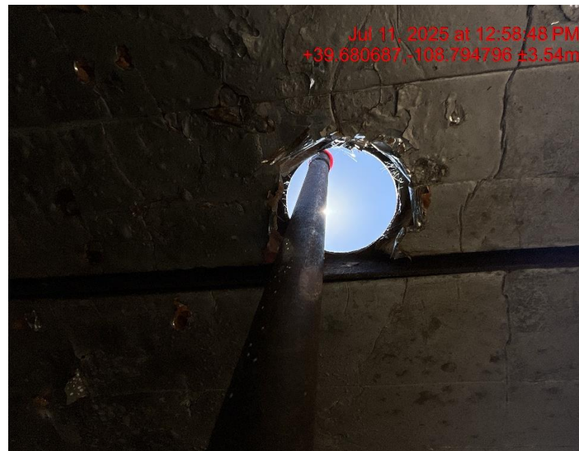
Photo # 9729 Hole in separator building/wildlife hazard/available for entry by wildlife
