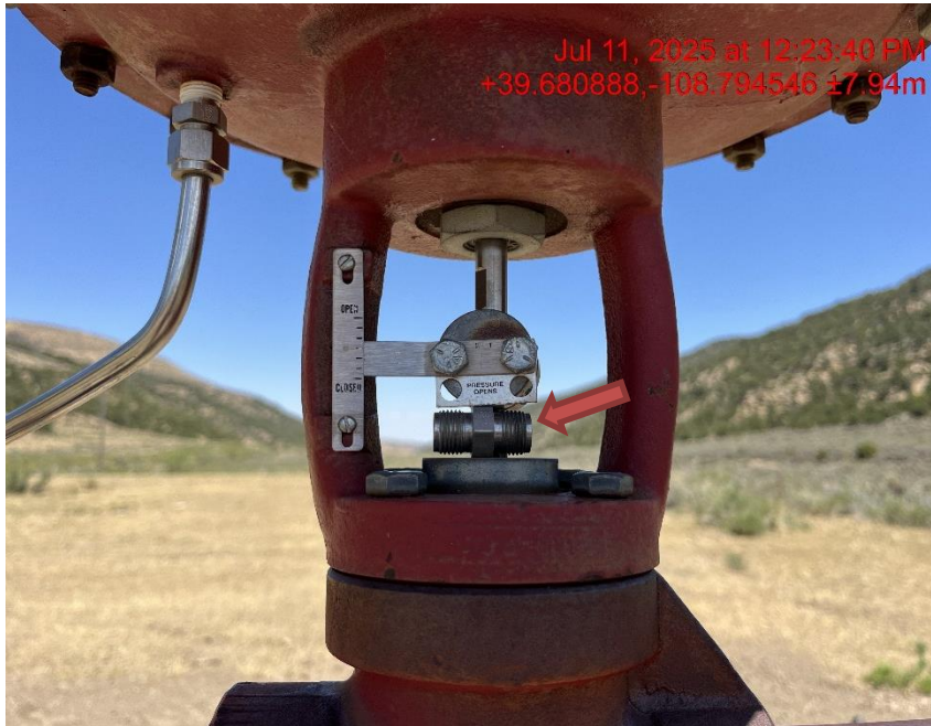
Photo # 9697 Equipment has been modified and is not being operated in a safe manner
