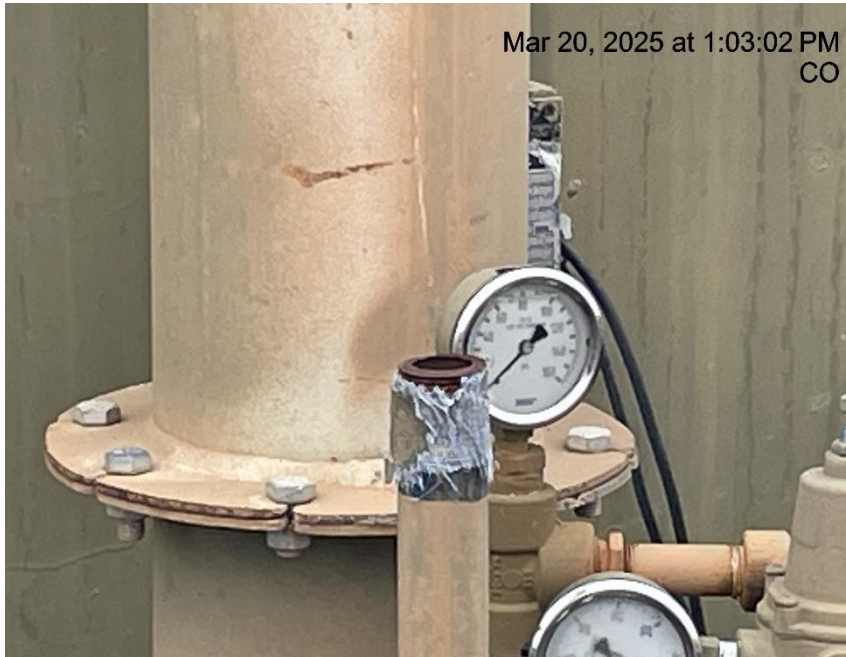
Photo # 5856 From inspection 708906068 conducted on 03/20/2025 PRV vent line does not comply with CECMC pressure safety device rules
