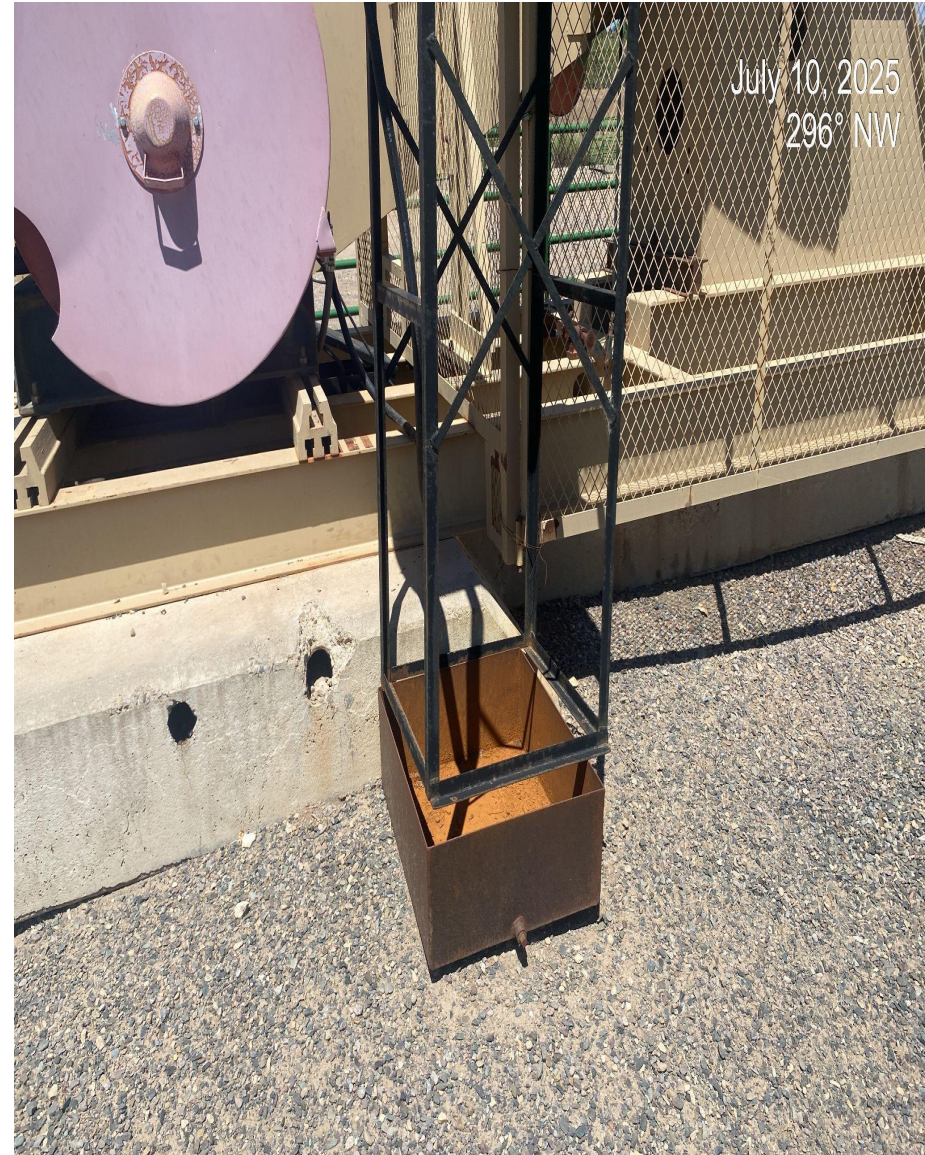
Photo 3. Lube tank secondary containments at both pump jacks have no wildlife cover/protections.
