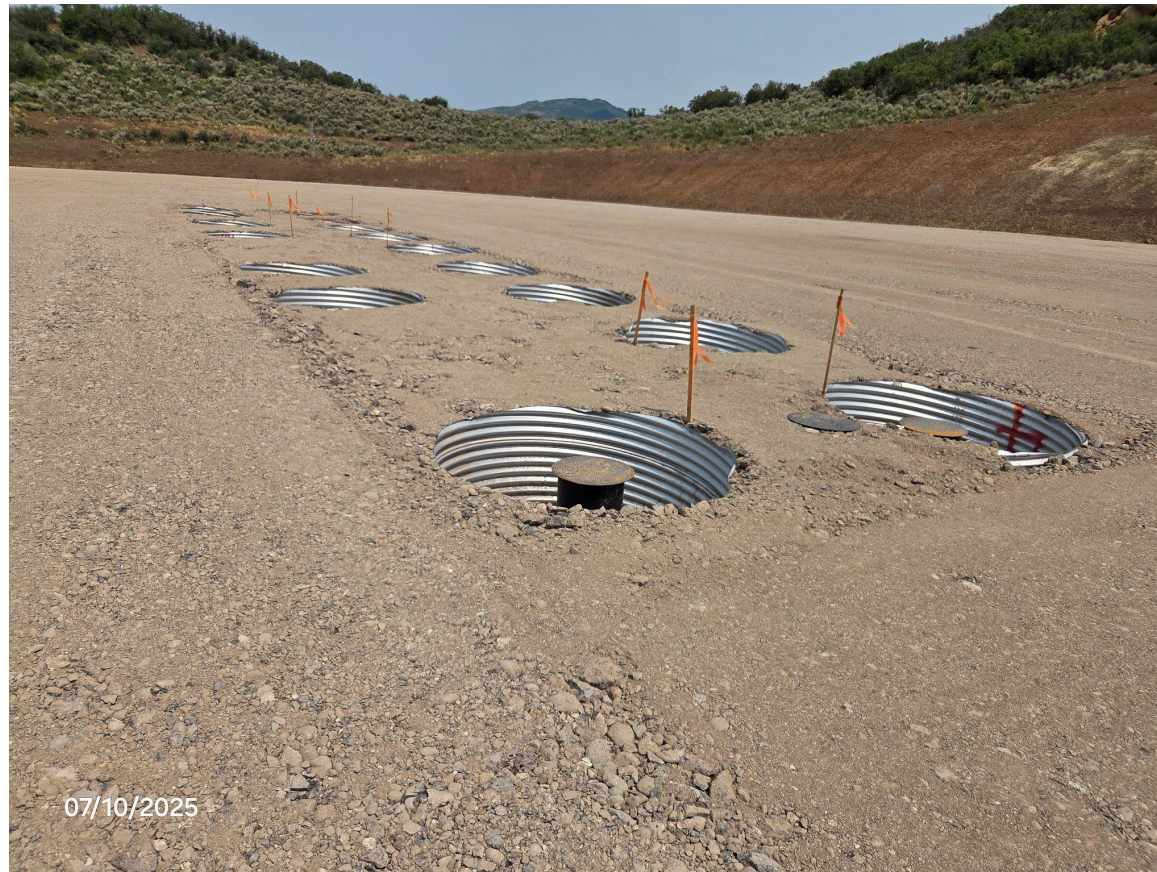
Photo 20: Photo shows cellars are missing required covers/fence.
