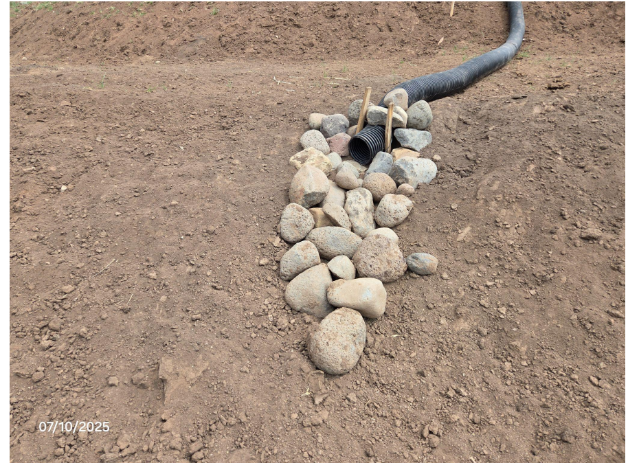
Photo 17: Slope drain outlets on the southwest end of the Location. See comments under photo 15.
