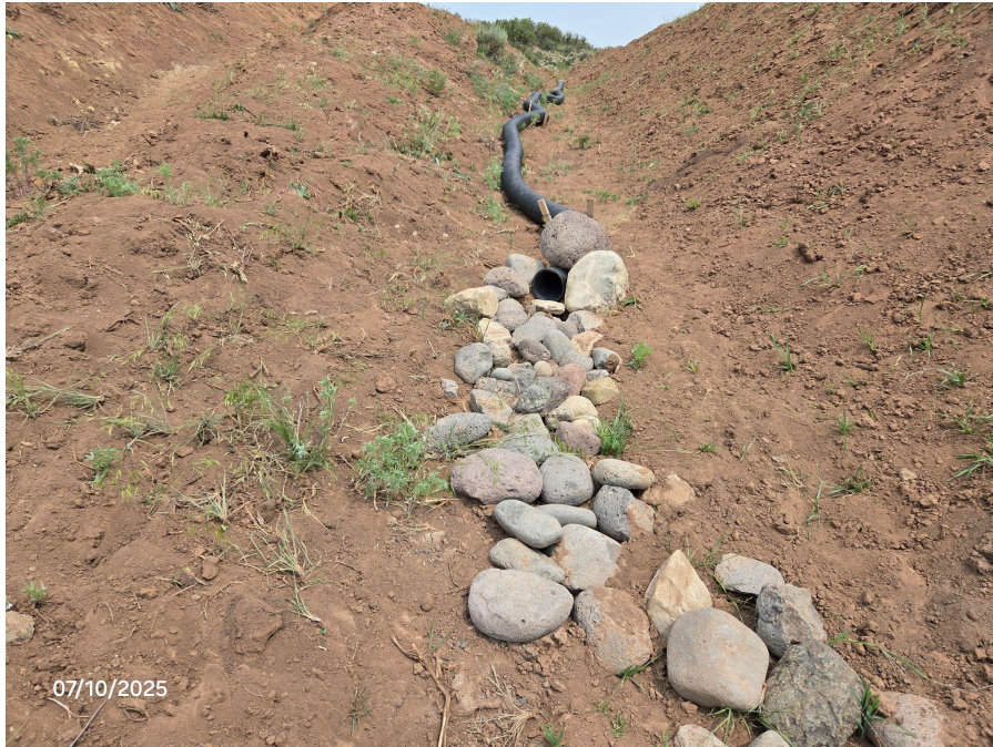
Photo 17: Slope drain outlets on the southwest end of the Location. See comments under photo 15.
