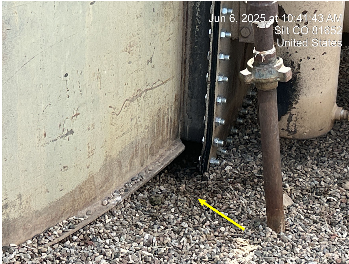
Photo 5: Photo shows a chipmunk burrow at the bottom of a tank battery. Maintenance is advised.
