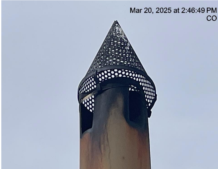
Photo # 6184 From inspection/audit 708906074 conducted on 03/20/2025 Bird protection on separator insufficient /burner stack available for entry by wildlife/wildlife hazard
