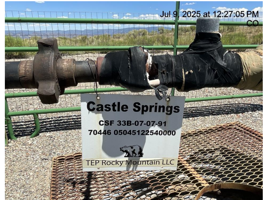
Photo # 296 Wellhead sign lacks required information
