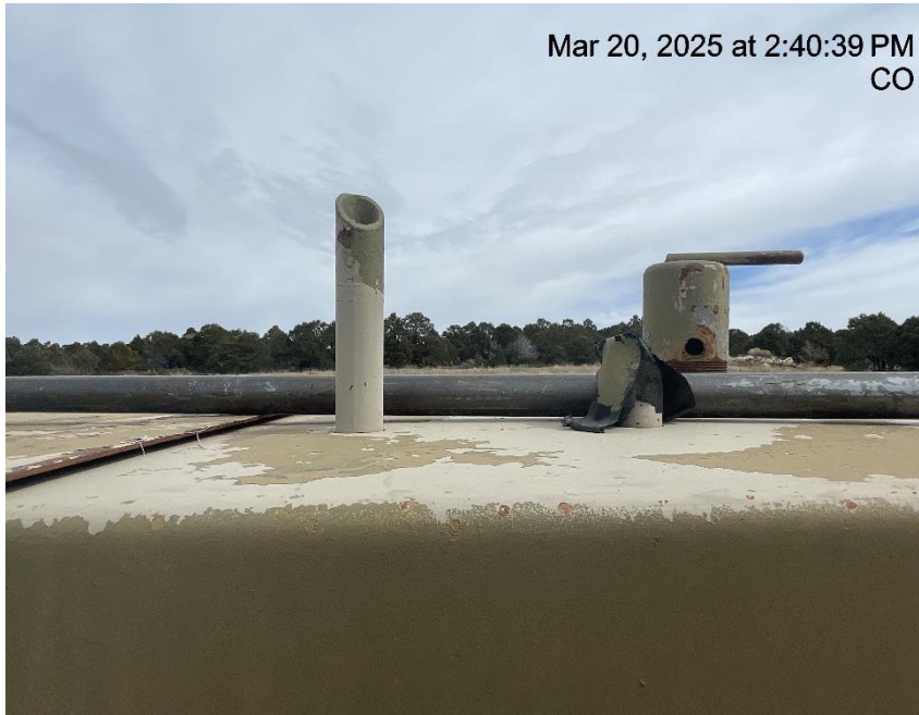
Photo # 6182 From inspection/audit 708906074 conducted on 03/20/2025 PRV vent line on separator does not comply with CECMC pressure safety device rules
