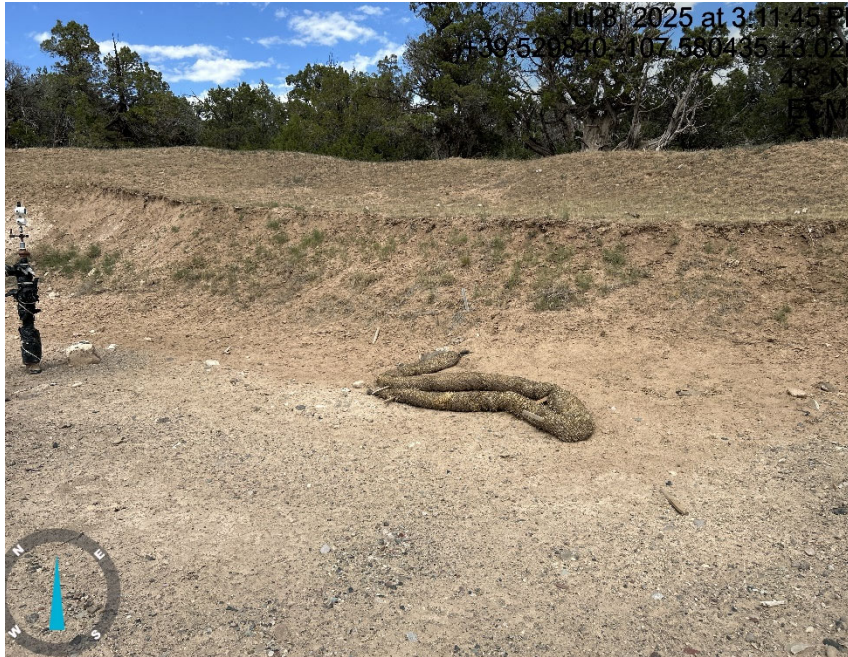
Cut slope erosion and waddles are debris
