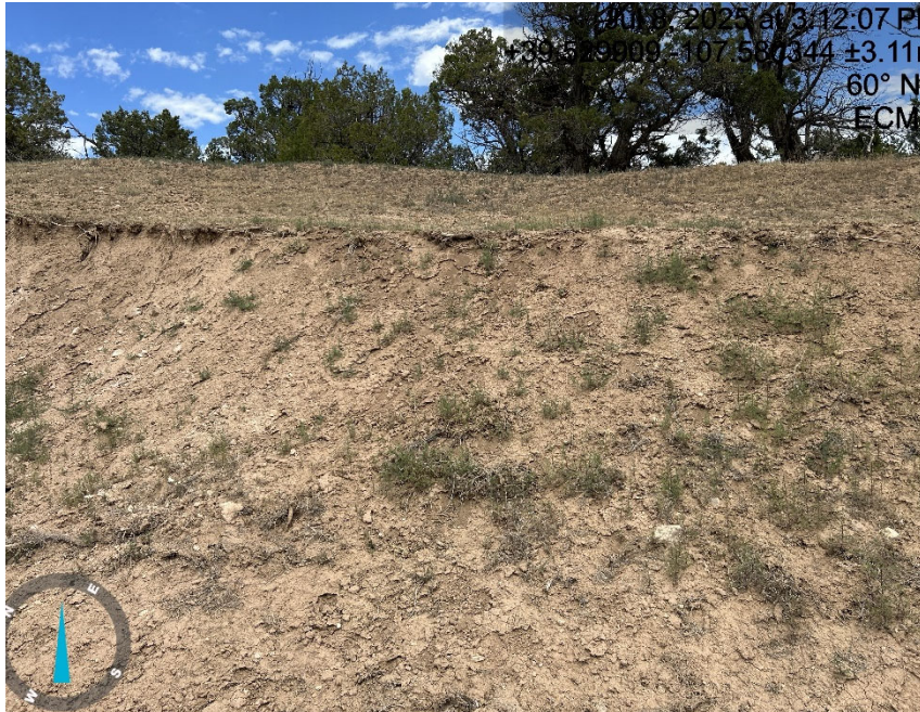
Cut slope erosion and waddles are debris
