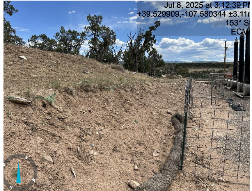
Cut slope erosion and waddles are debris
