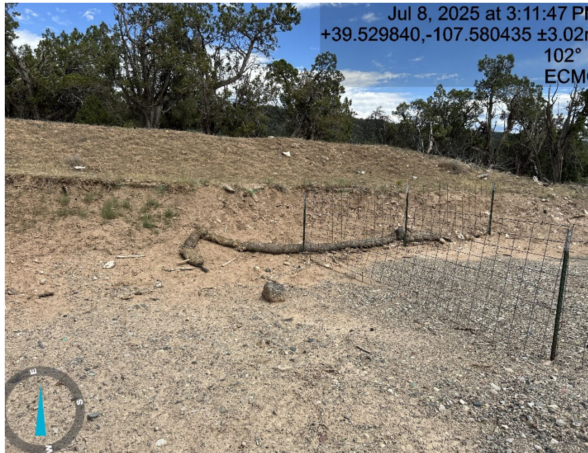
Cut slope erosion and waddles are debris
