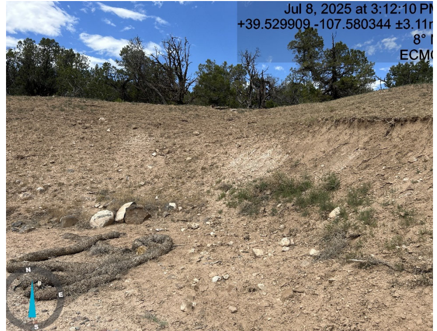
Cut slope erosion and waddles are debris
