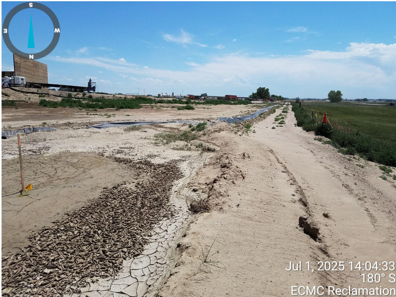
Photo 19. Photo taken west of the northwestern perimeter of location, facing South. Photo illustrates the Operator has failed to implement perimeter stormwater control BMPs.
