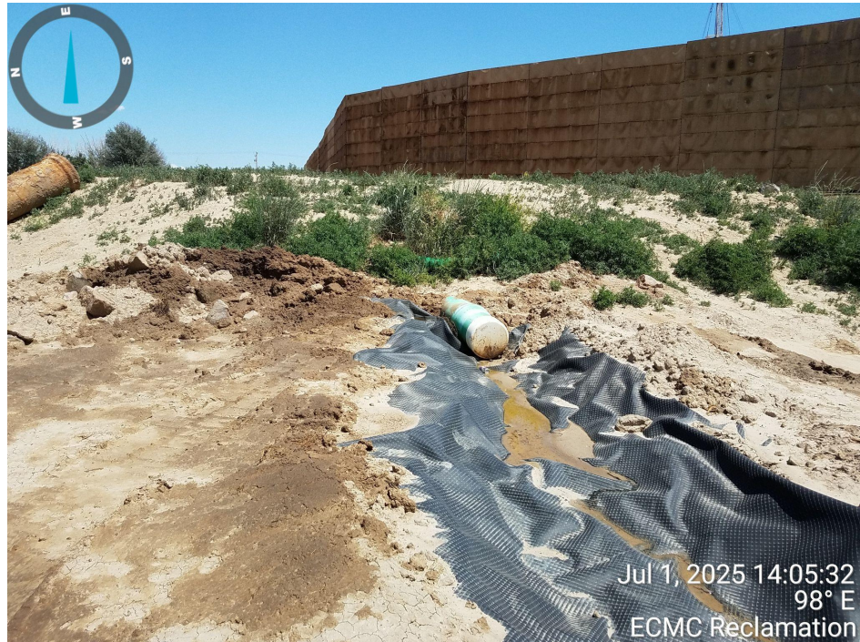
Photo 18. Photo taken from the PVC standpipe outlet, facing East. Photo illustrates the outlet has been capped to prevent the discharge of E&P waste mixed with stormwater discharge.
