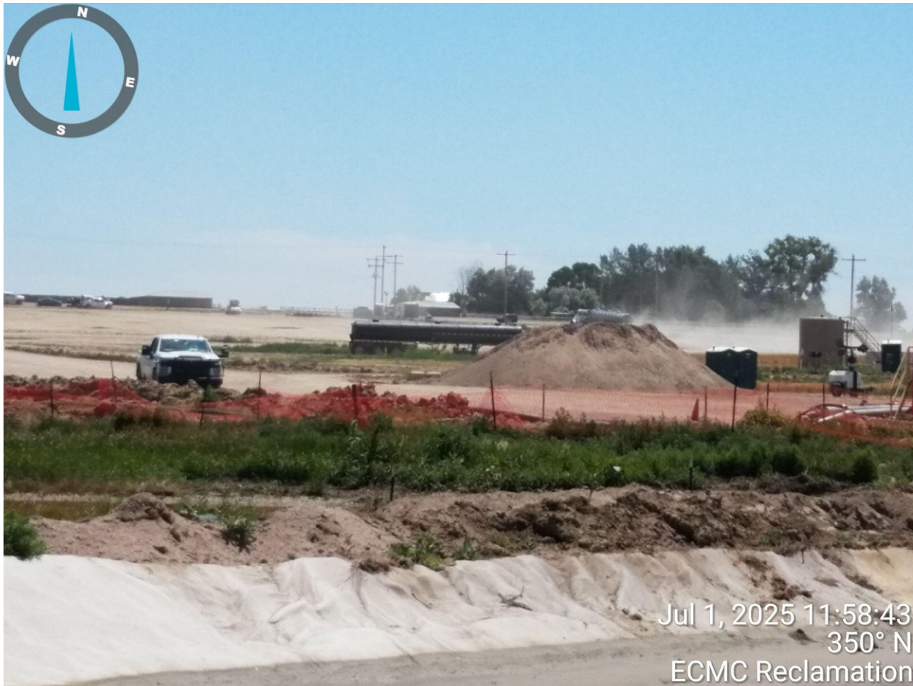
Photo 4. Photo taken from an Operator service truck along a portion of the main location access road, facing East. Photo illustrates fugitive dust from the service truck which needs to be controlled.
