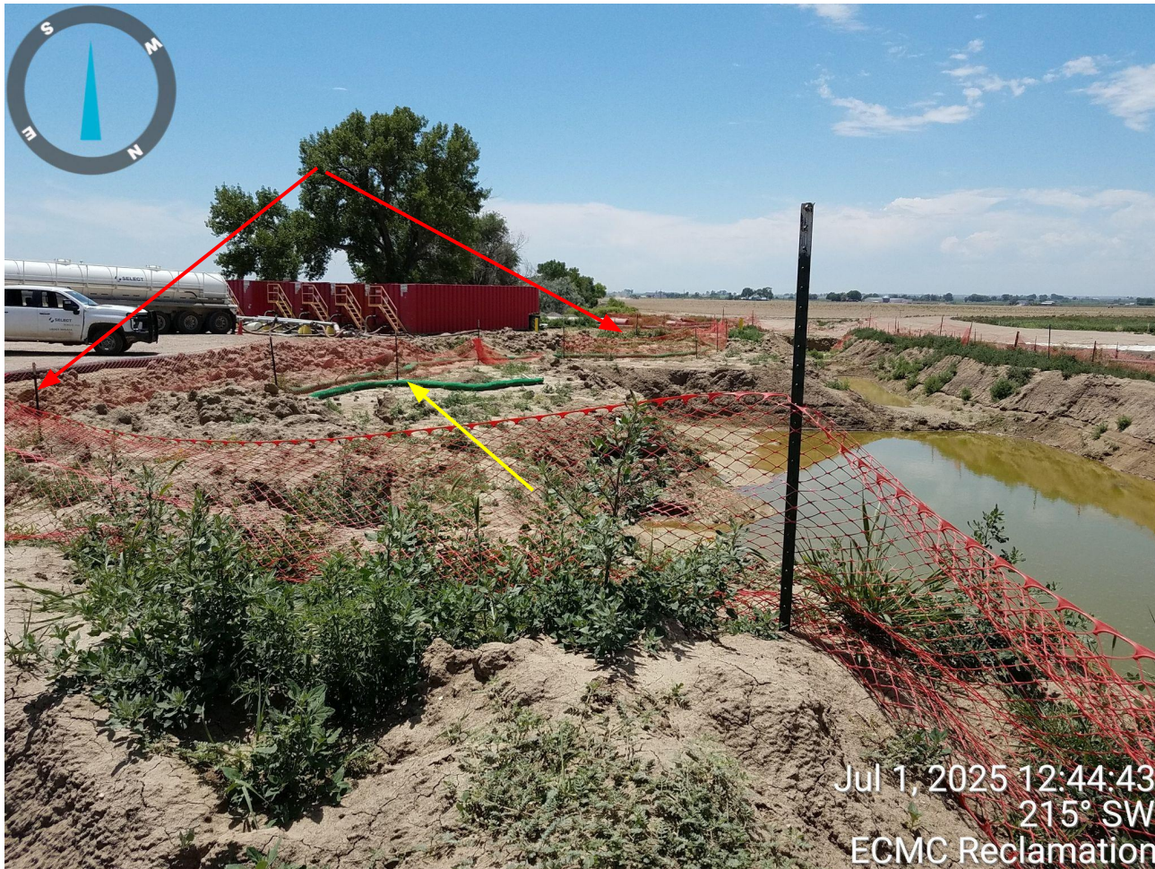
Photo 6. Photo taken from the southern emergency pit, facing South. Operator has a filtrex BMP along portions of the interior unconsolidated berm material that are not in proper functioning condition (yellow arrow) but no BMP along the exterior unconsolidated berm material (red arrows).
