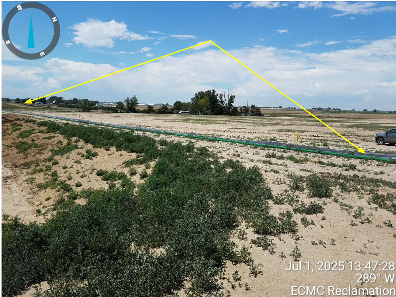
Photo 15. Photo taken from the northeastern perimeter of location, facing Northwest. Photo illustrates filter wattle BMPs (yellow arrows) have been installed along an irrigation ditch and appear to be in proper functioning condition.
