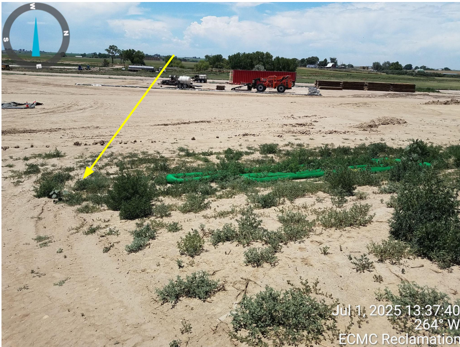
Photo 11. Photo taken from the southwestern perimeter of location along the topsoil stockpile, facing West. Photo illustrates Operator has failed to implement perimeter stormwater BMPs for the topsoil stockpile (yellow arrow).
