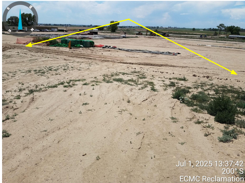
Photo 12. Photo taken from the southwestern perimeter of location along the topsoil stockpile, facing South. Photo illustrates stormwater erosion along the topsoil stockpile without implementing perimeter stormwater BMPs for the topsoil stockpile (yellow arrows).
