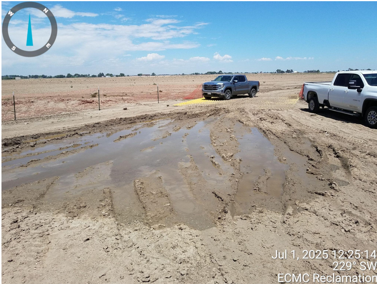
Photo 2. Photo taken from the entrance of the Greeley #2 Canal road, facing North. Photo illustrates what appears to be stormwater run-on from County Road 70. Operator has a vehicle tracking device BMP in need of maintenance (yellow mat); however, this BMP alone is not sufficient to prevent vehicle track out onto County Road 70.
