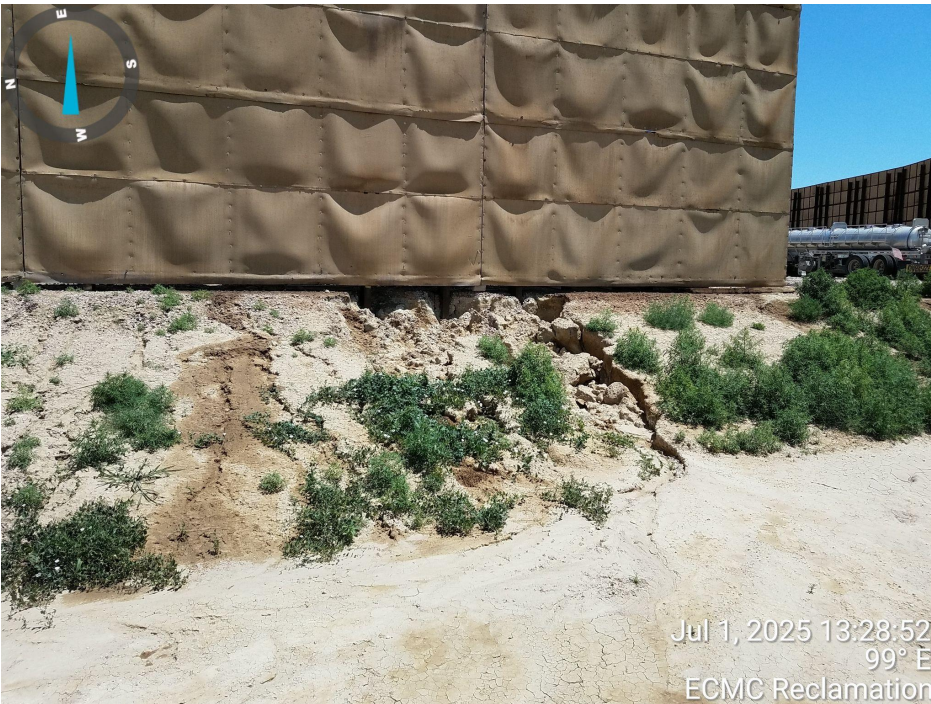
Photo 9. Photo taken from the southwestern fill slope of location, facing East. Photo illustrates gully erosion that was believed to be caused by the initial incident back in April 2025 per information from an Operator representative. Operator has failed to conduct stormwater repairs.
