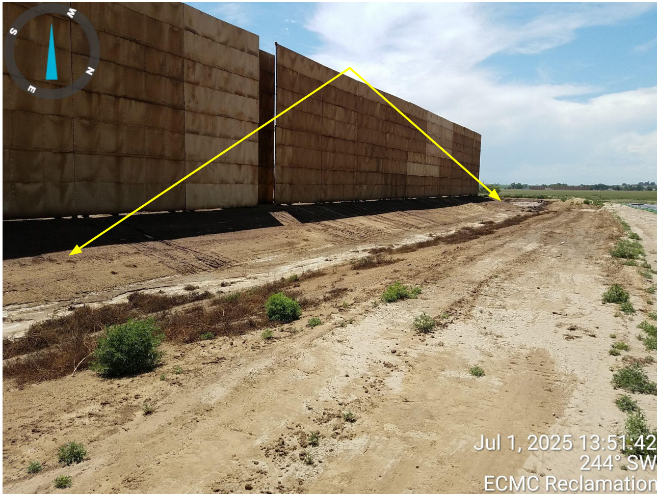
Photo 16. Photo taken from the northern fill slope of location, facing West. Photo illustrates rill erosion that was believed to be caused by the initial incident back in April 2025 per information from an Operator representative. Operator has failed to conduct stormwater repairs.
