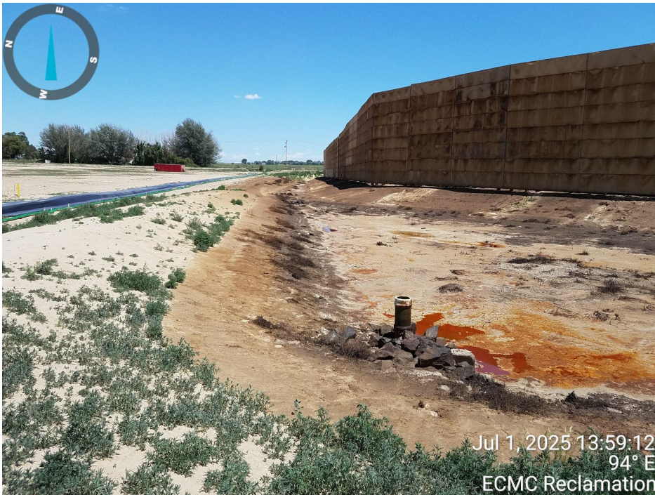
Photo 17. Photo taken from the northeastern perimeter of location, facing East. Photo illustrates a detention pond with impacted material. The PVC standpipe outlet has been capped. See Photo 18.
