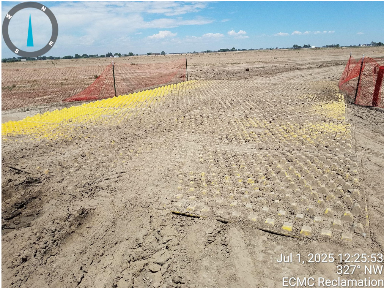
Photo 3. Close up photo taken from the vehicle tracking device BMP in need of maintenance (yellow mat).
