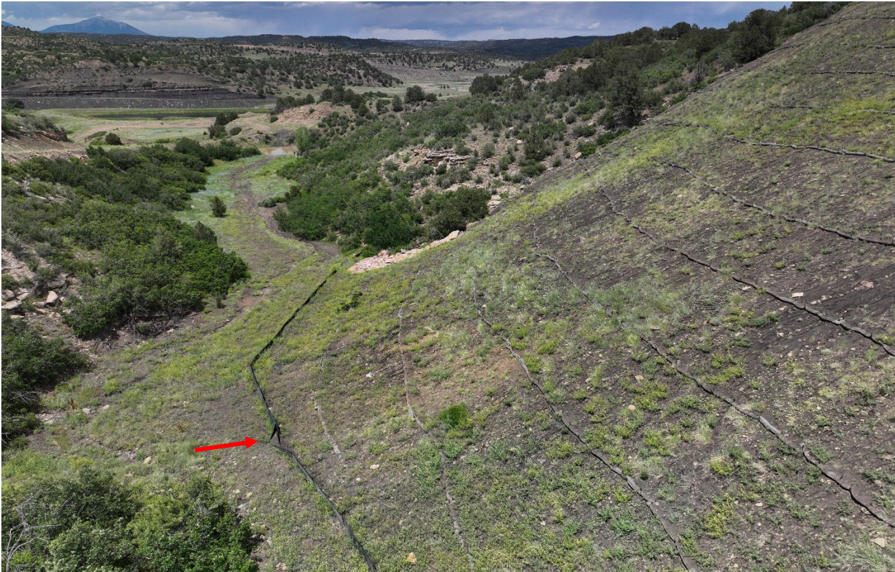
Photo 9. Facing north along the bottom of the fill slope. It appears the silt fence needs maintenance at red arrow.
