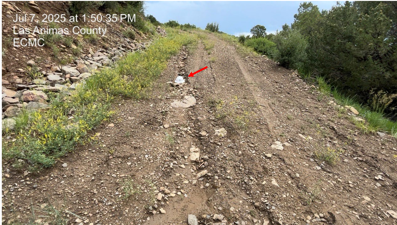
Photo 1. Facing south along the access road. There is erosion along the road. Red arrow points to a hard hat in the erosion channel for scale.
