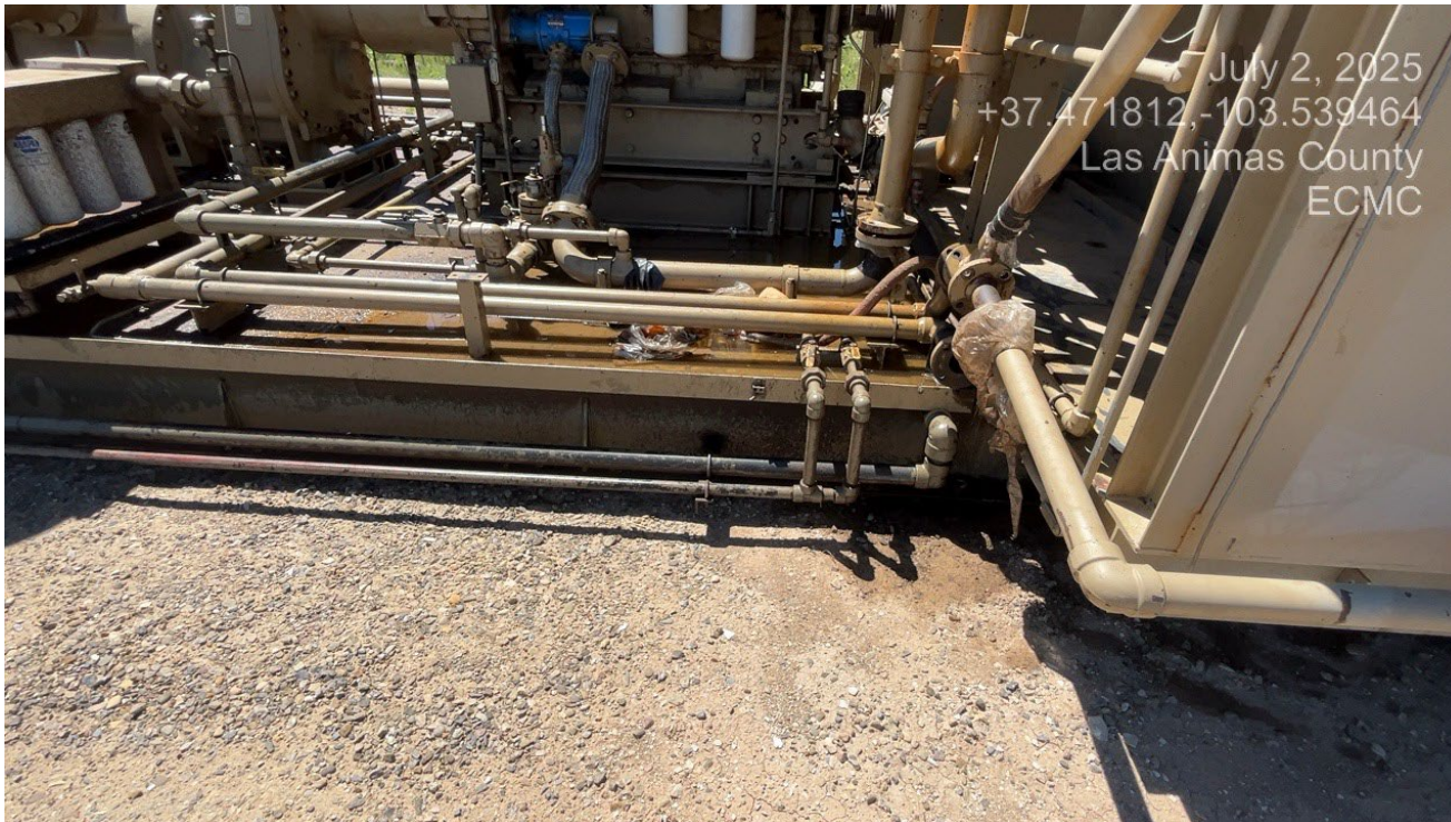
Photo 5. There is some fluids that are staining the soil. Oily fluids need to be cleaned up and properly disposed.
