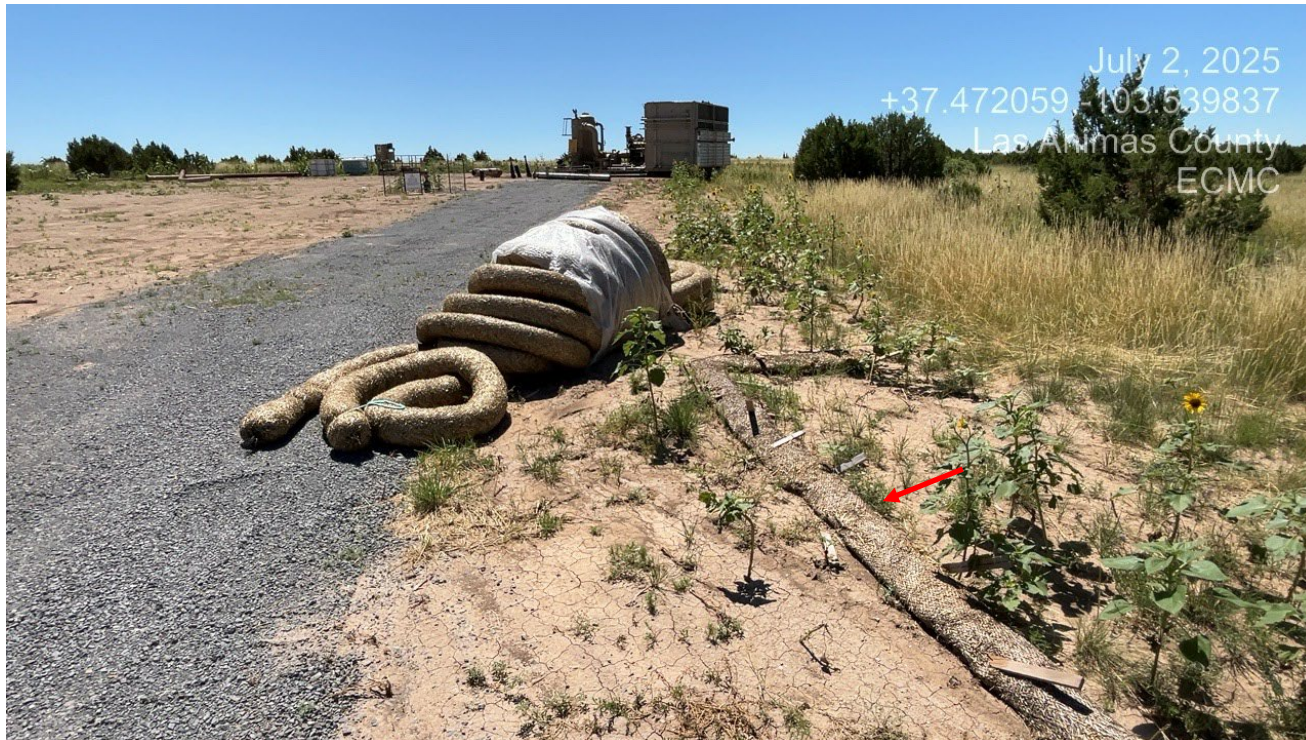
Photo 2. Facing southeast toward the location. There are a pile of wattles partly in the road. There are degraded wattles shown at red arrow.
