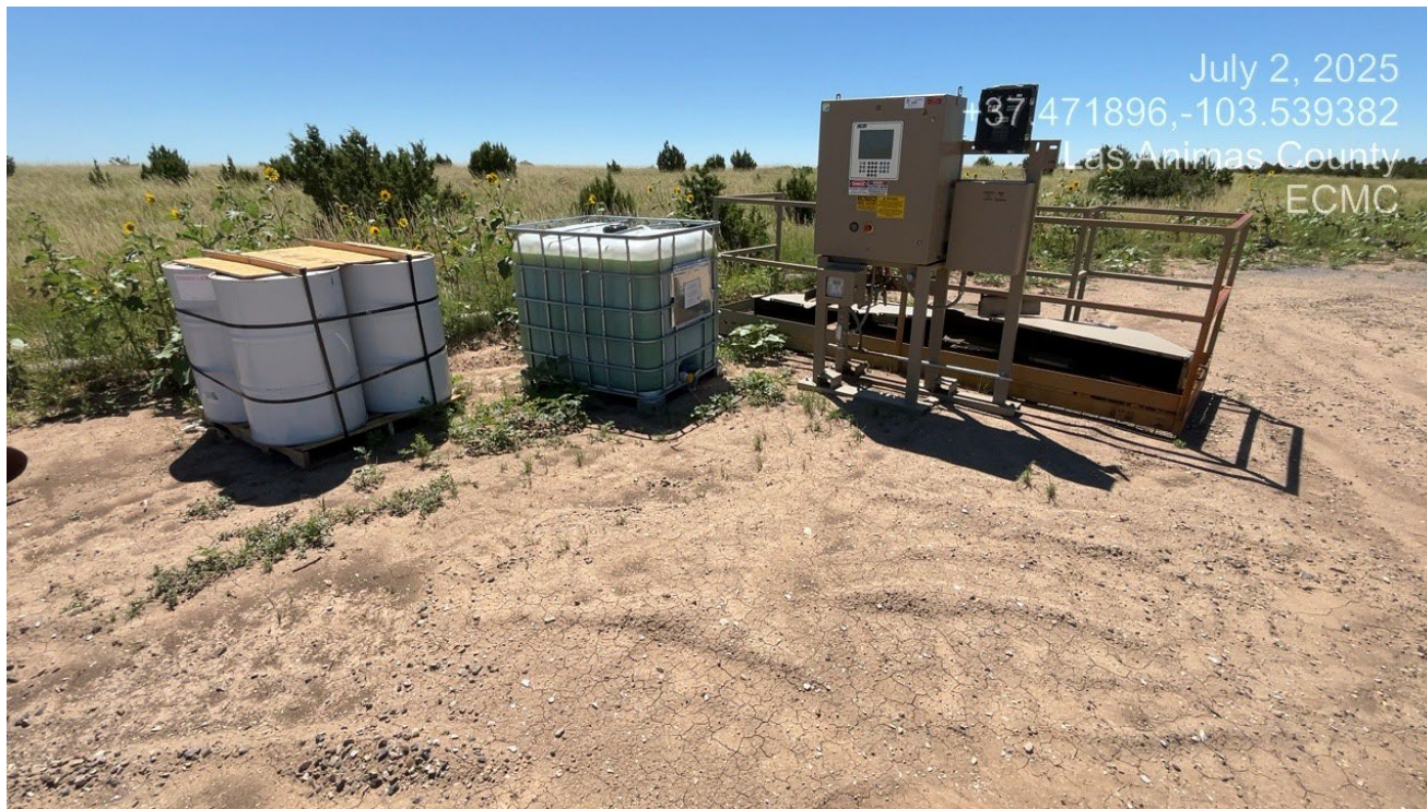
Photo 6. There are chemical barrels stored on location. Secondary containment will need to be implemented.
