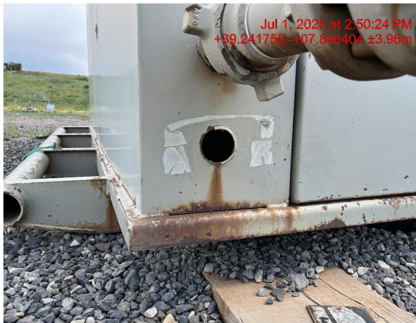
Photo # 9379 Hole in separator building/wildlife hazard/available for entry by wildlife
