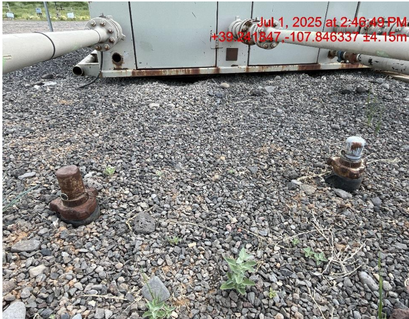
Photo # 9373 Multiple unused flowlines do not comply with CECMC 600 & 1100 series rules
