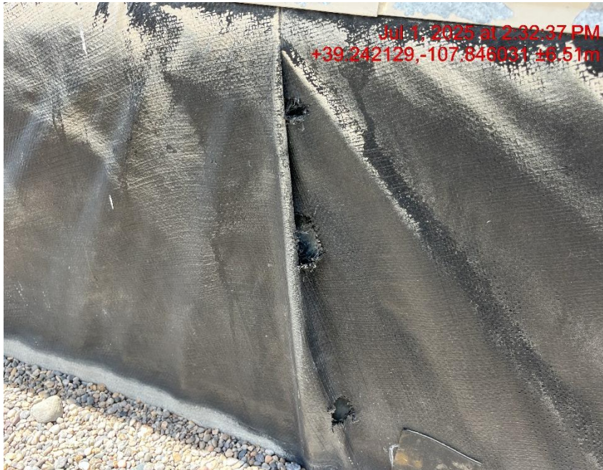
Photo # 9347 Multiple holes in secondary containment liner/liner needs maintenance
