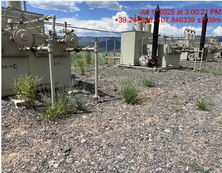
Photo # 9387 Weeds/undesirable plant species surrounding production equipment constitutes a fire hazard
