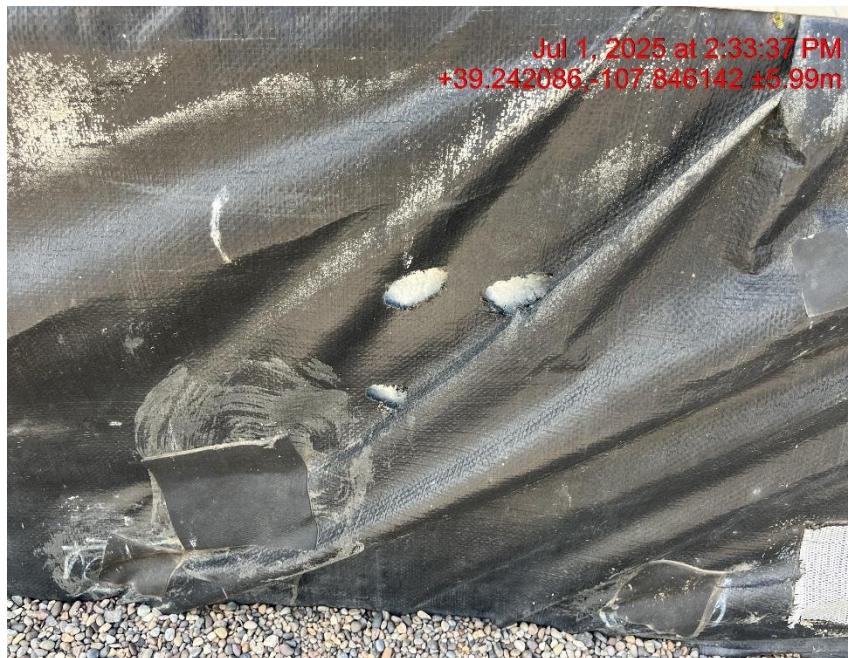
Photo # 9355 Multiple holes in secondary containment liner/liner needs maintenance
