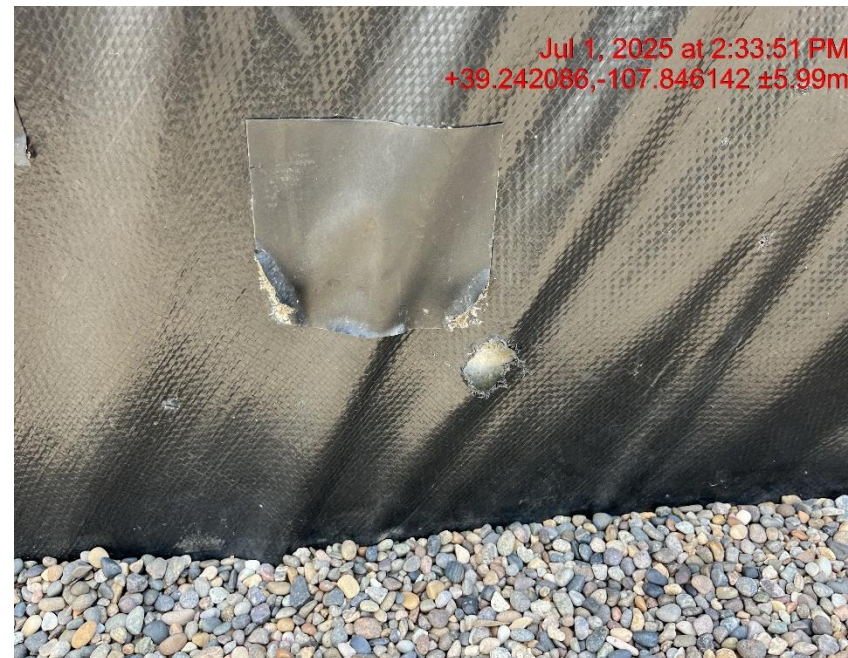
Photo # 9356 Multiple holes in secondary containment liner/liner needs maintenance
