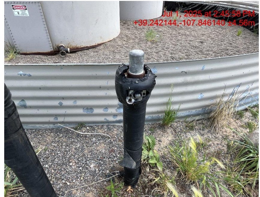
Photo # 9372 Unused flowline does not comply with CECMC 600 & 1100 series rules
