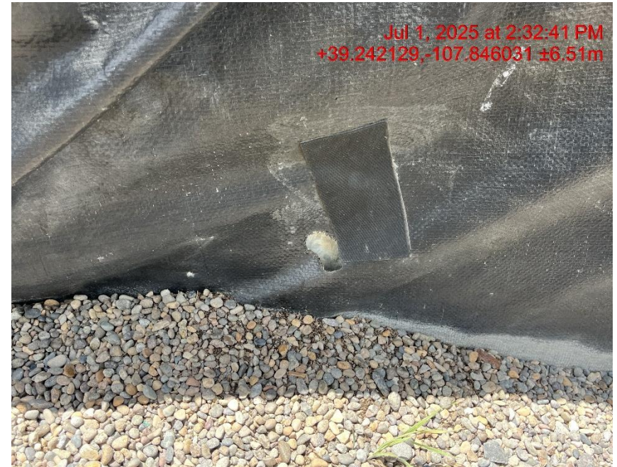
Photo # 9348 Multiple holes in secondary containment liner/liner needs maintenance
