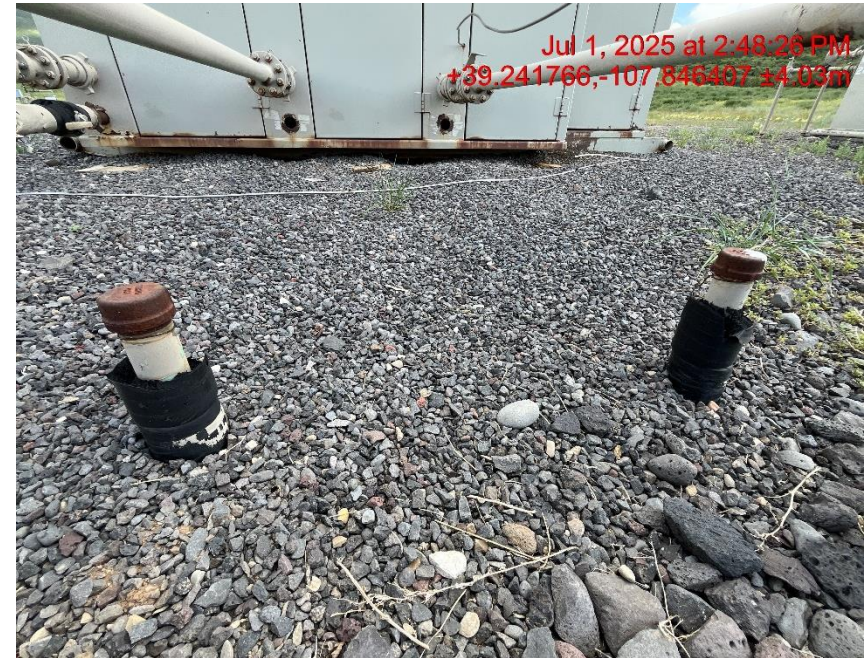
Photo # 9374 Multiple unused flowlines do not comply with CECMC 600 & 1100 series rules
