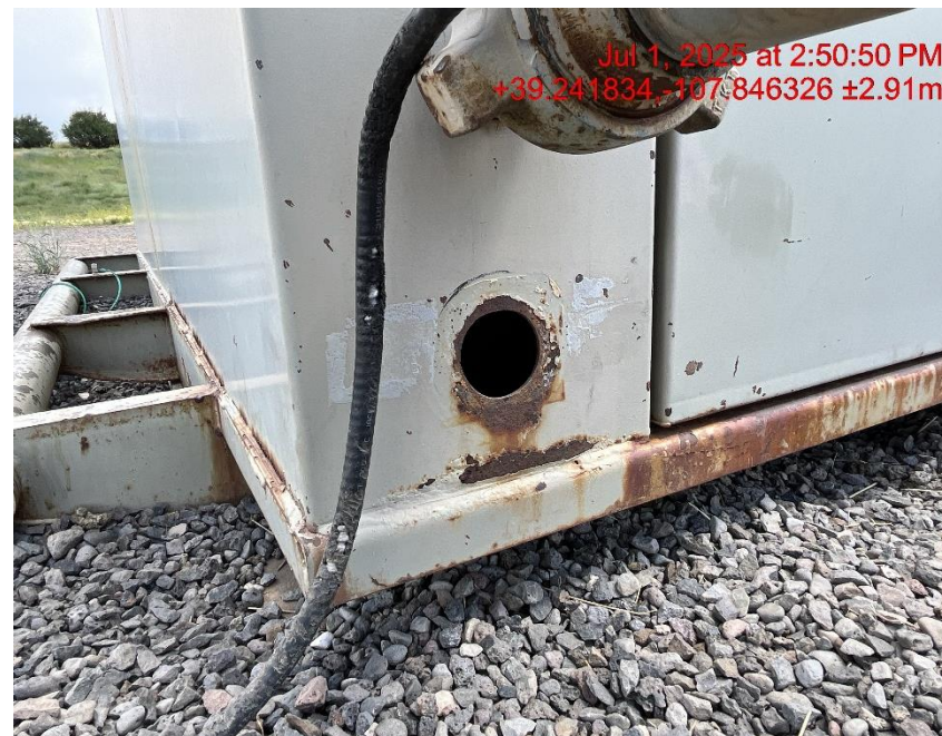
Photo # 9380 Hole in separator building/wildlife hazard/available for entry by wildlife
