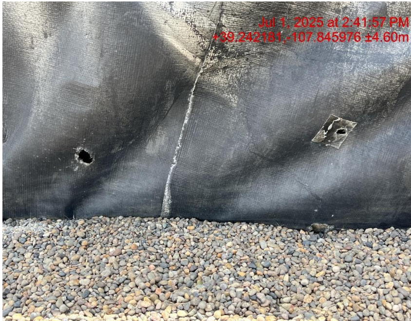
Photo # 9367 Multiple holes in secondary containment liner/liner needs maintenance
