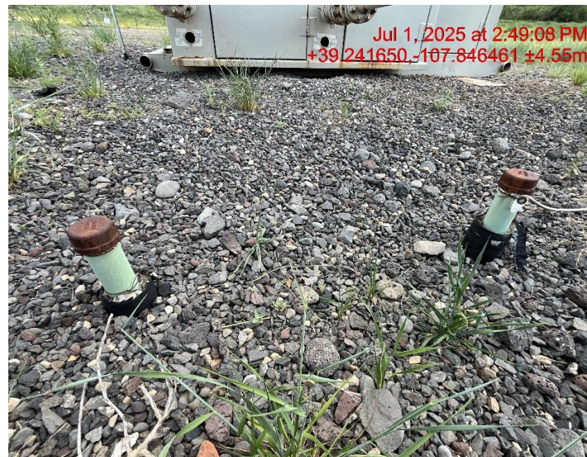
Photo # 9376 Multiple unused flowlines do not comply with CECMC 600 & 1100 series rules
