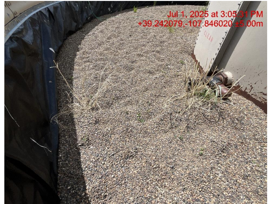
Photo # 9399 Weeds/undesirable plant species surrounding production equipment constitutes a fire hazard
