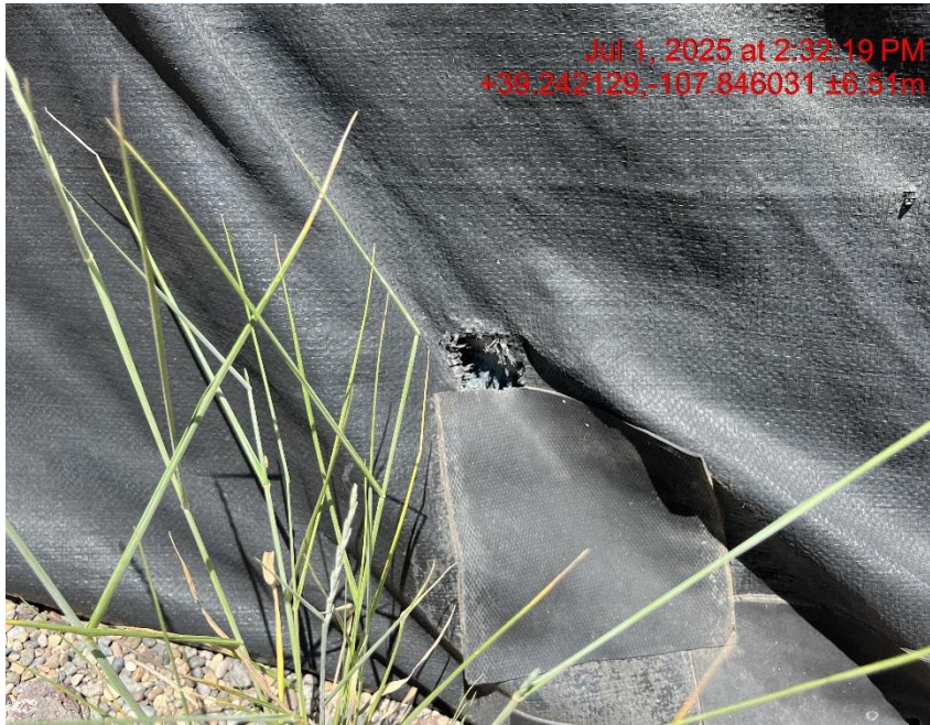
Photo # 9345 Multiple holes in secondary containment liner/liner needs maintenance
