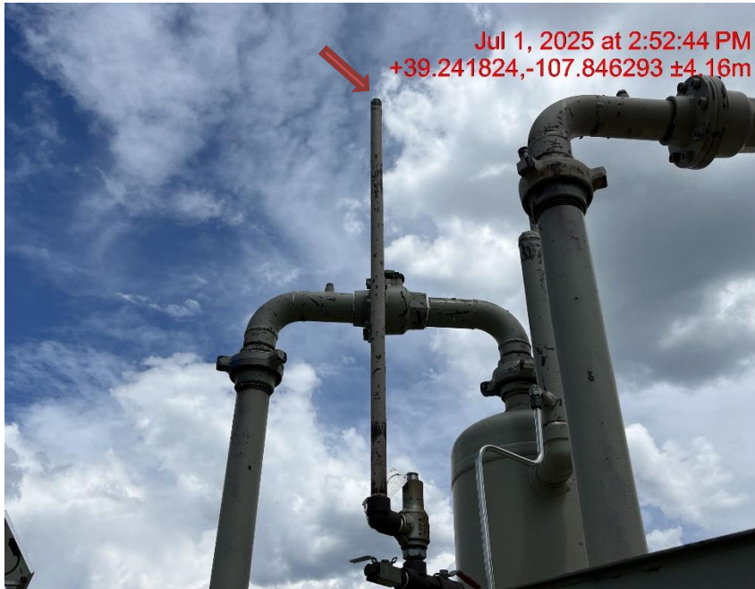
Photo # 9381 PRV vent line does not comply with CECMC pressure safety device rules
