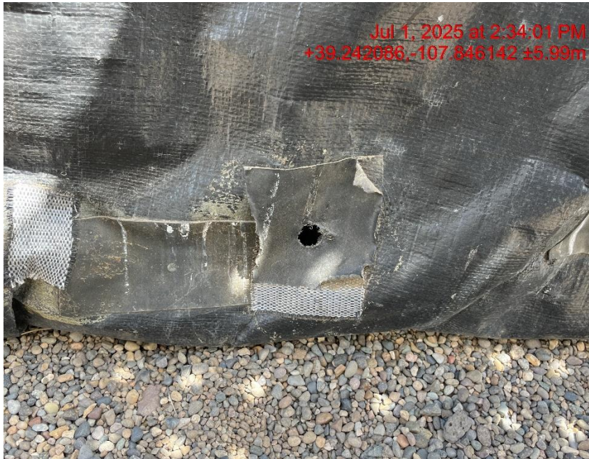
Photo # 9357 Multiple holes in secondary containment liner/liner needs maintenance
