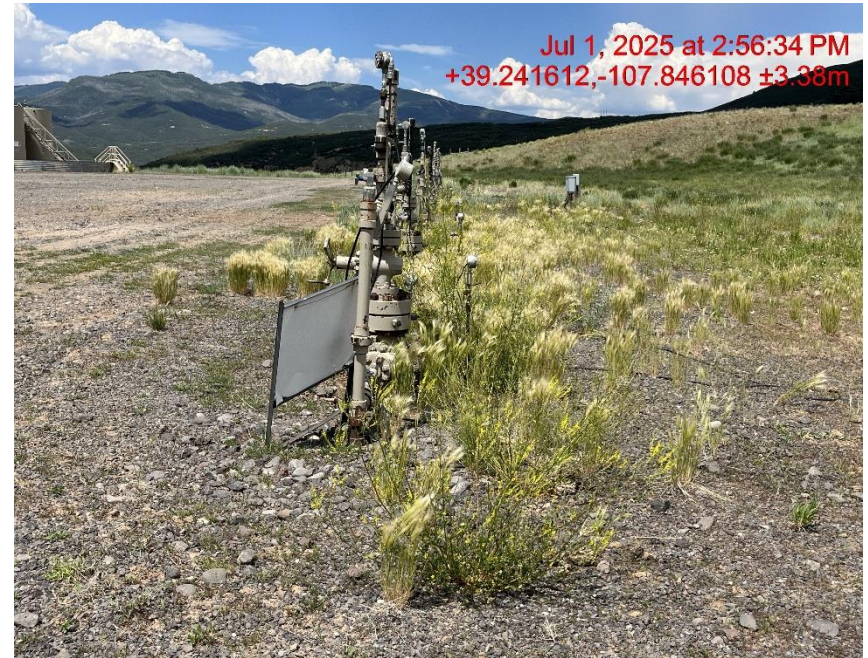
Photo # 9384 Weeds/undesirable plant species surrounding production equipment constitutes a fire hazard
