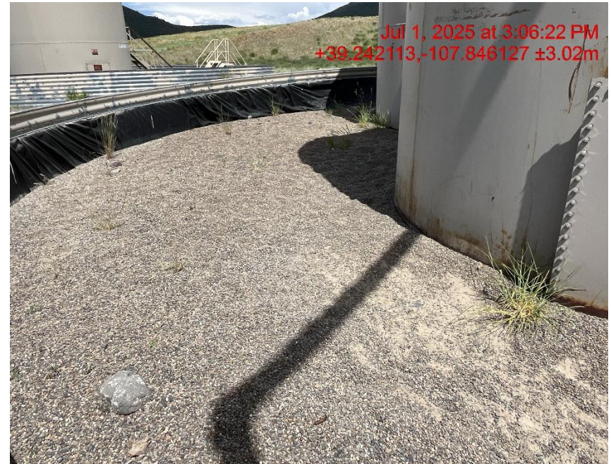
Photo # 9401 Weeds/undesirable plant species surrounding production equipment constitutes a fire hazard
