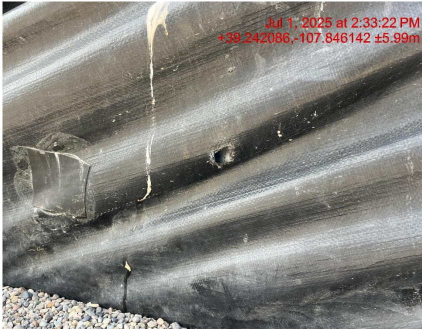
Photo # 9353 Multiple holes in secondary containment liner/liner needs maintenance
