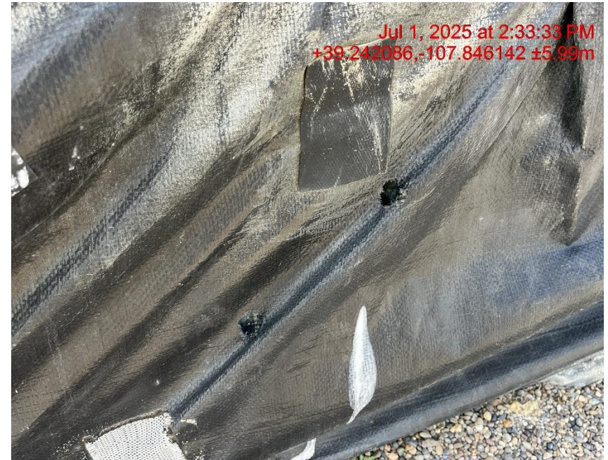
Photo # 9354 Multiple holes in secondary containment liner/liner needs maintenance
