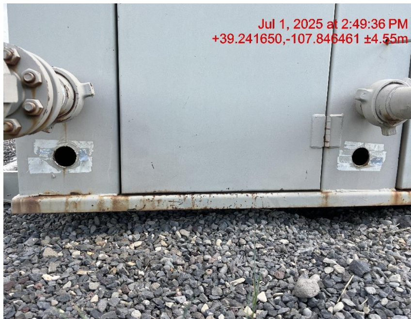
Photo # 9377 Multiple holes in separator buildings open to wildlife/ available for entry by wildlife
