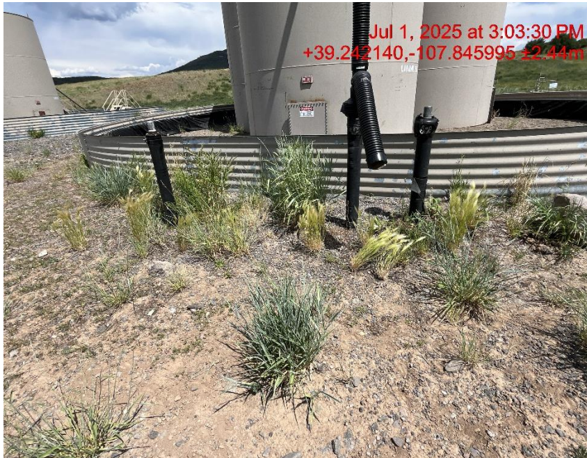
Photo # 9395 Weeds/undesirable plant species surrounding production equipment constitutes a fire hazard
