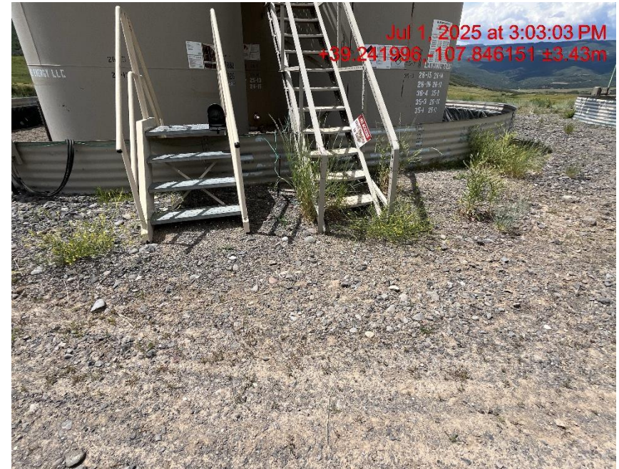
Photo # 9393 Weeds/undesirable plant species surrounding production equipment constitutes a fire hazard
