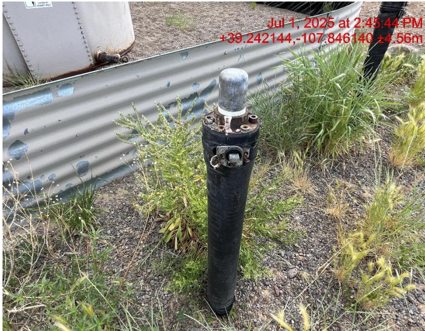
Photo # 9371 Unused flowline does not comply with CECMC 600 & 1100 series rules
