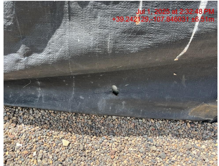
Photo # 9350 Multiple holes in secondary containment liner/liner needs maintenance
