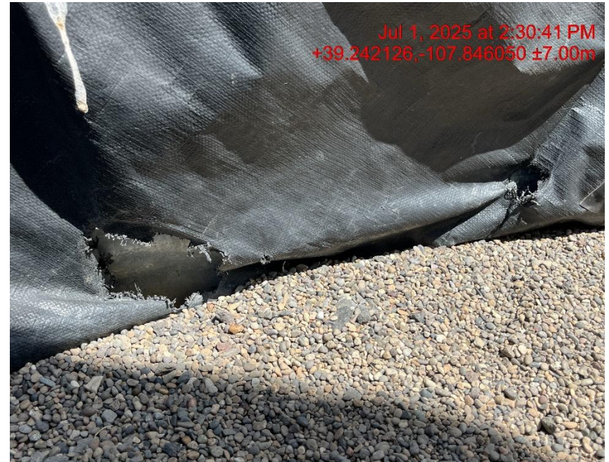
Photo # 9343 Multiple holes in secondary containment liner/liner needs maintenance
