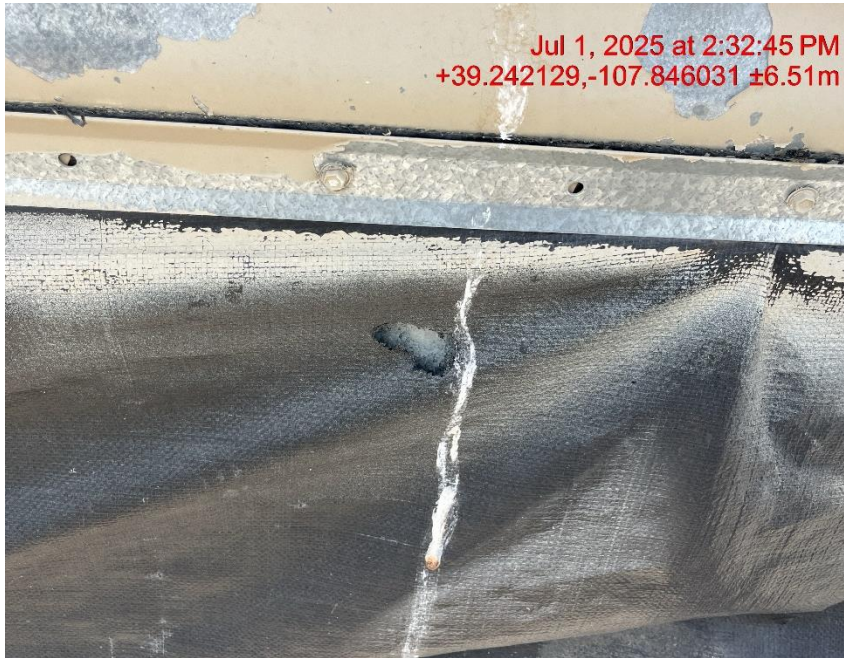
Photo # 9349 Multiple holes in secondary containment liner/liner needs maintenance
