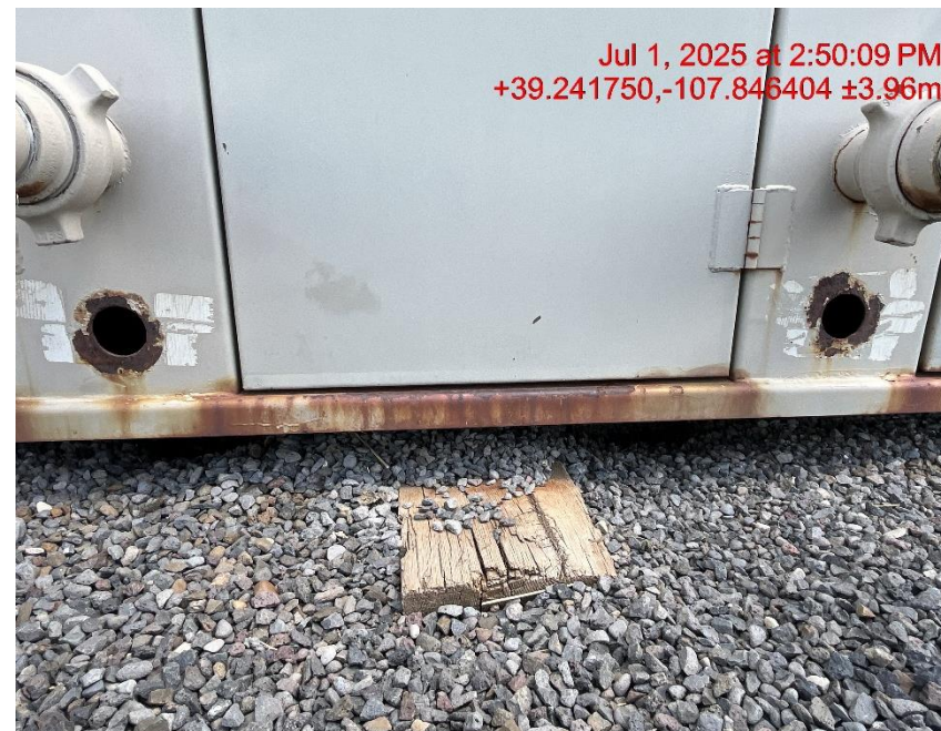
Photo # 9378 Multiple holes in separator buildings open to wildlife/ available for entry by wildlife
