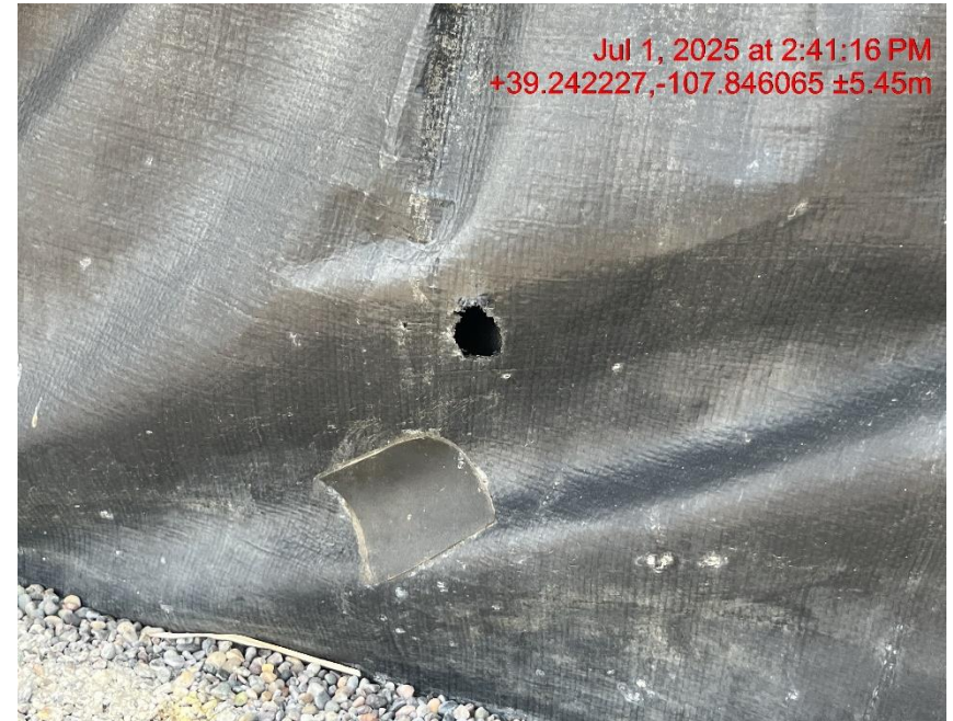
Photo # 9366 Multiple holes in secondary containment liner/liner needs maintenance
