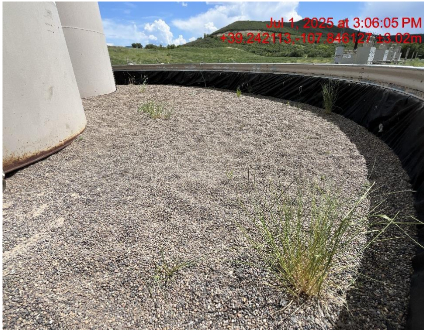
Photo # 9400 Weeds/undesirable plant species surrounding production equipment constitutes a fire hazard
