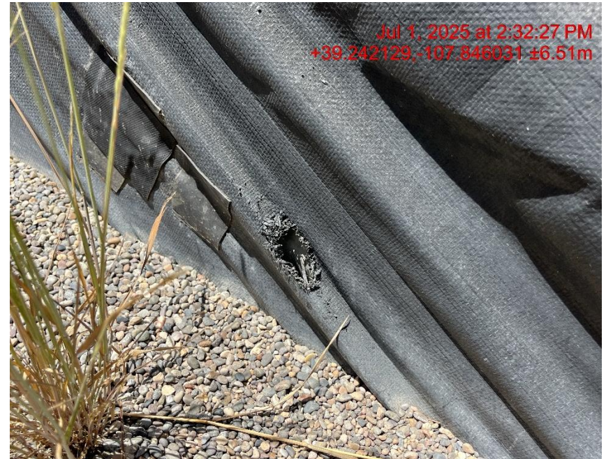
Photo # 9346 Multiple holes in secondary containment liner/liner needs maintenance
