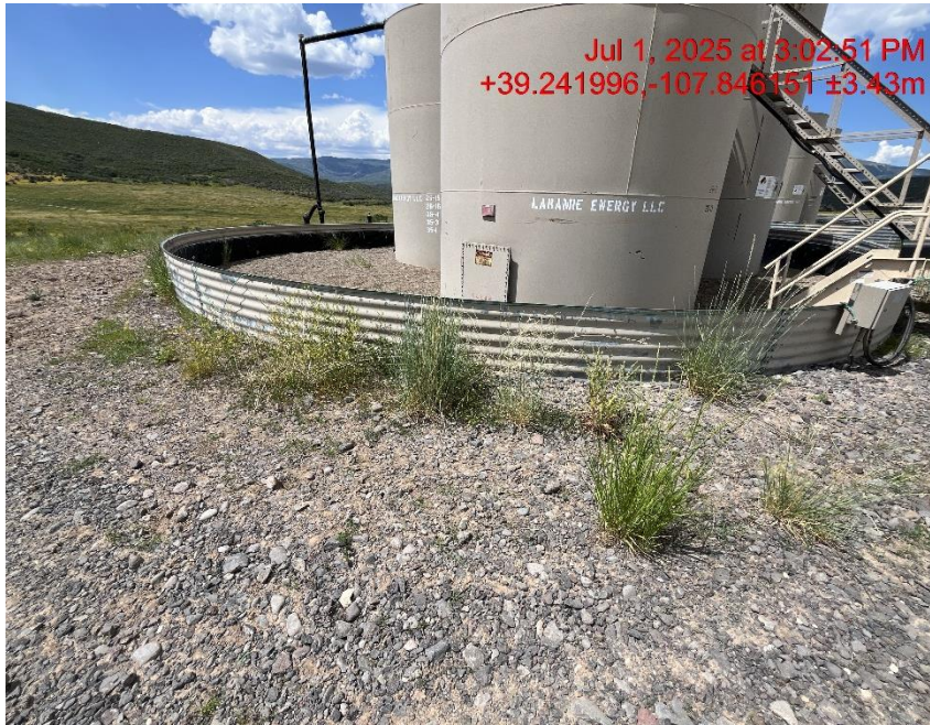
Photo # 9392 Weeds/undesirable plant species surrounding production equipment constitutes a fire hazard
