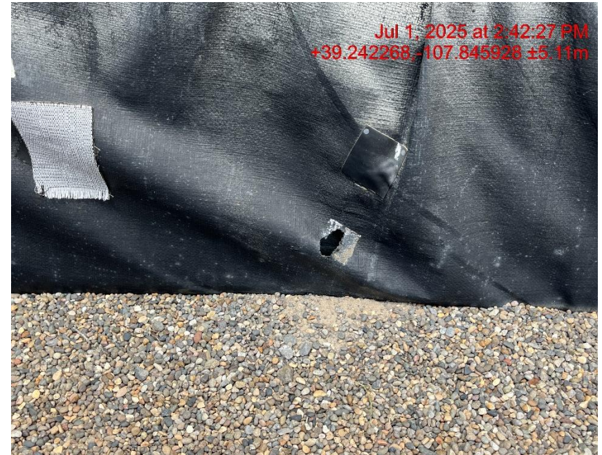
Photo # 9368 Multiple holes in secondary containment liner/liner needs maintenance
