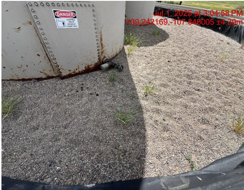
Photo # 9398 Weeds/undesirable plant species surrounding production equipment constitutes a fire hazard
