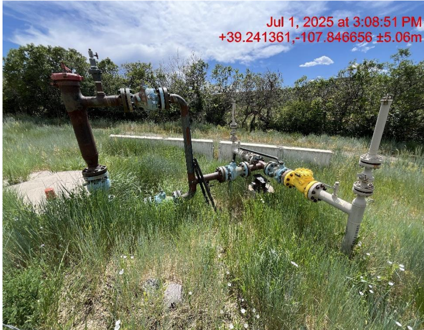
Photo # 9402 Location - Weeds/undesirable plant species surrounding production equipment constitutes a fire hazard
