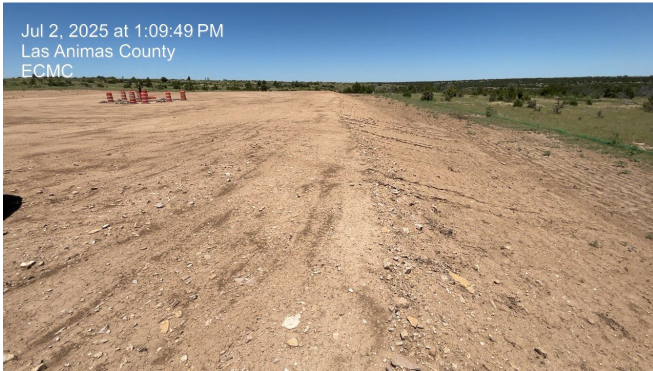
Photo 4. There is erosion beginning to occur along the fill slope of the location.
