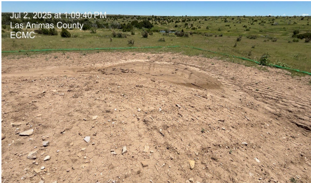
Photo 5. Facing southwest corner of the location. The sediment trap has filled in with sediment and needs maintenance.
