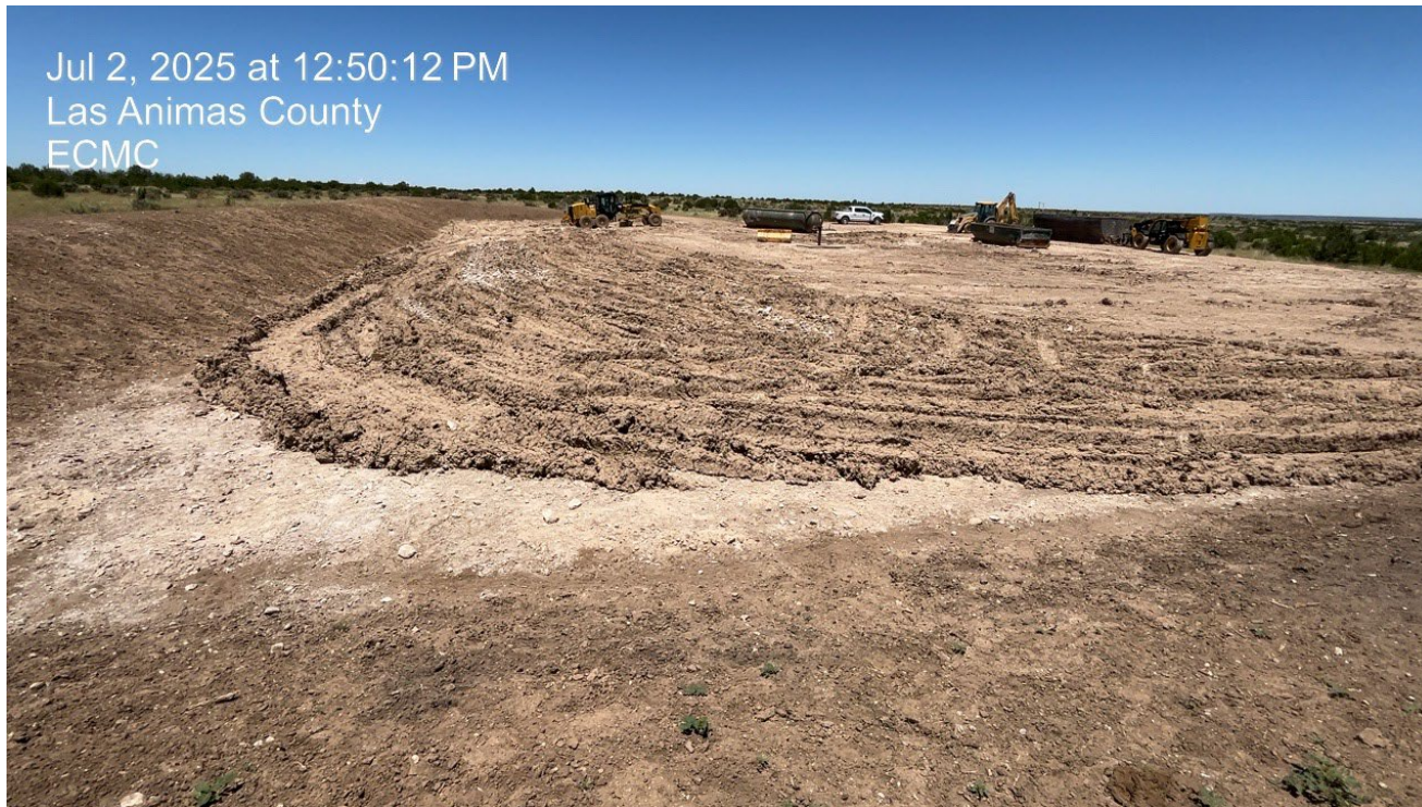
Photo 9. Facing northeast at the location. The production area is not stabilized and there is vehicle tracking occurring.
