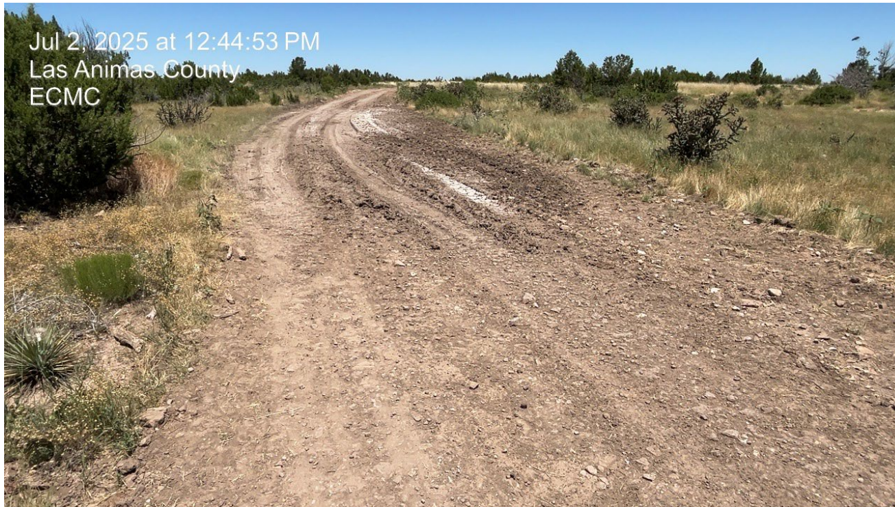
Photo 4. Facing north along the access road. Vehicles are driving outside of the road causing unnecessary disturbance. Vehicle tracking is occurring along the road.
