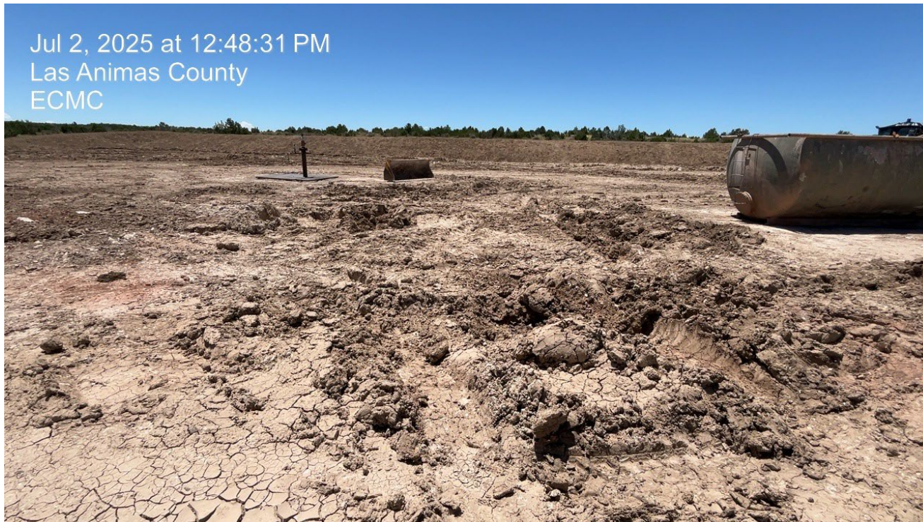
Photo 8. Facing west at the wellsite. The production area is not stabilized and there is vehicle tracking occurring.
