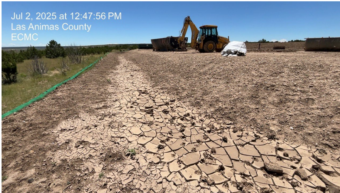
Photo 7. Facing south toward the east downhill perimeter. This ditch has filled in with sediment and needs to be cleaned out.
