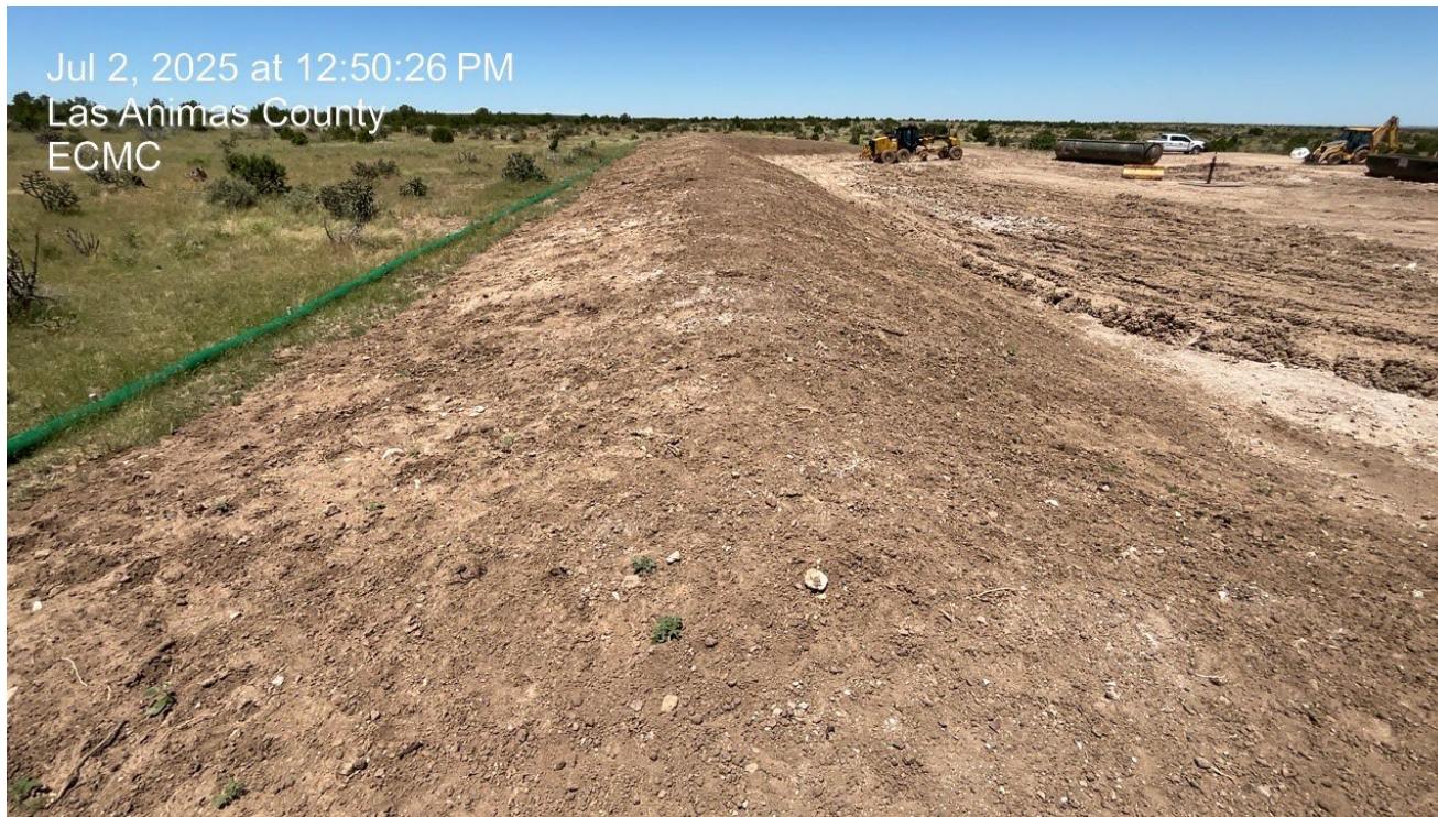
Photo 10. Facing north along the topsoil pile which needs to be seeded and stabilized.
