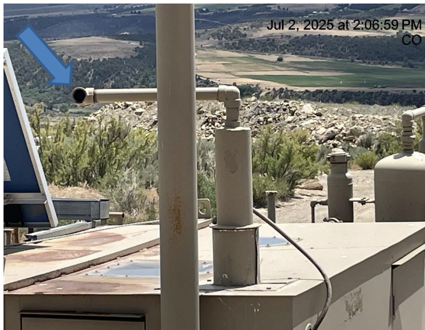
Photo # 9517 Open ended piping on separator/wildlife hazard/available for entry by wildlife
