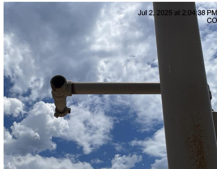
Photo # 9518 Open ended piping on separator/wildlife hazard/available for entry by wildlife
