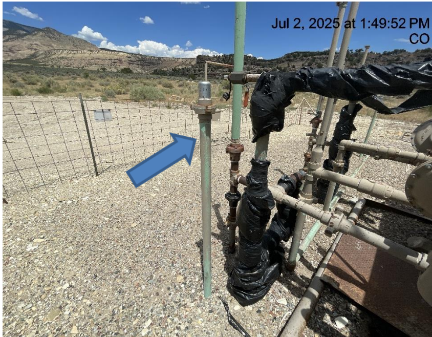
Photo # 9471 Unused flowline does not comply with CECMC rules
