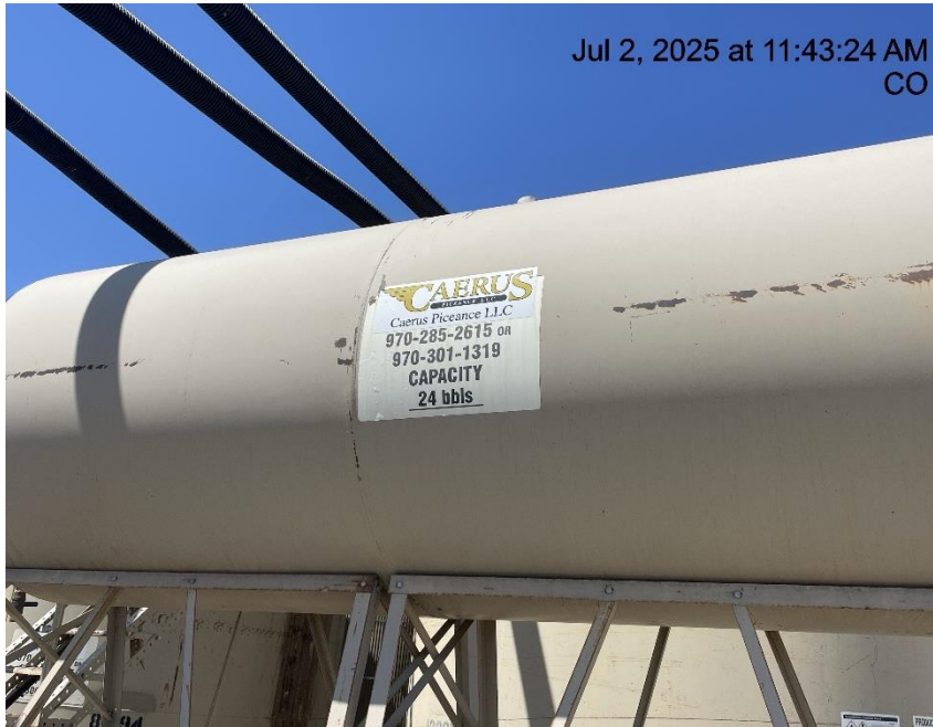
Photo # 9304 Methanol tank label contains inaccurate information
