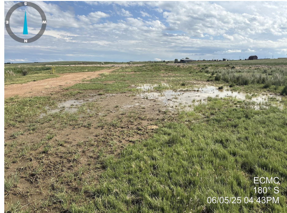
Photo 8. Photo taken of the tank battery location, facing South. Photo illustrates that vegetation has not established to Rule 1004 standards at the location.
