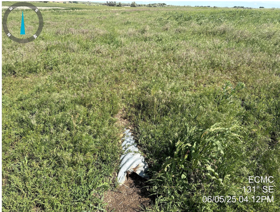
Photo 7. Photo taken of the access road to the well location, facing southeast. Photo illustrates that a partially-collapsed culvert remains on the access road.
