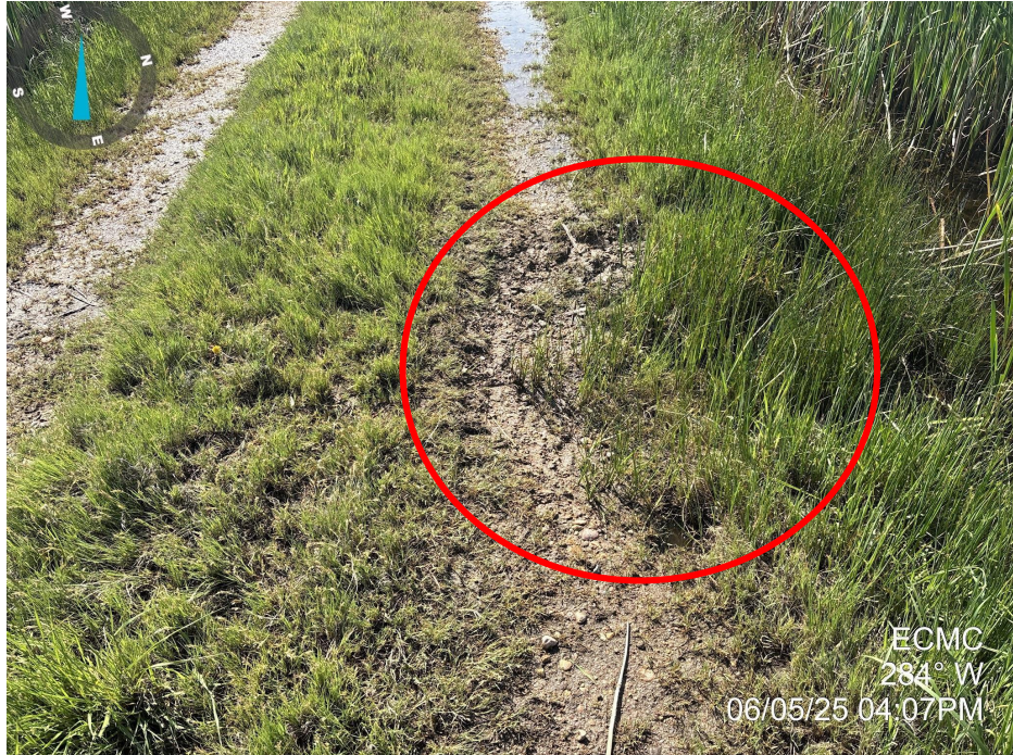
Photo 8. Photo taken of the access road. Photo illustrates stormwater erosion (highlighted in red circle) along a portion of the road.
