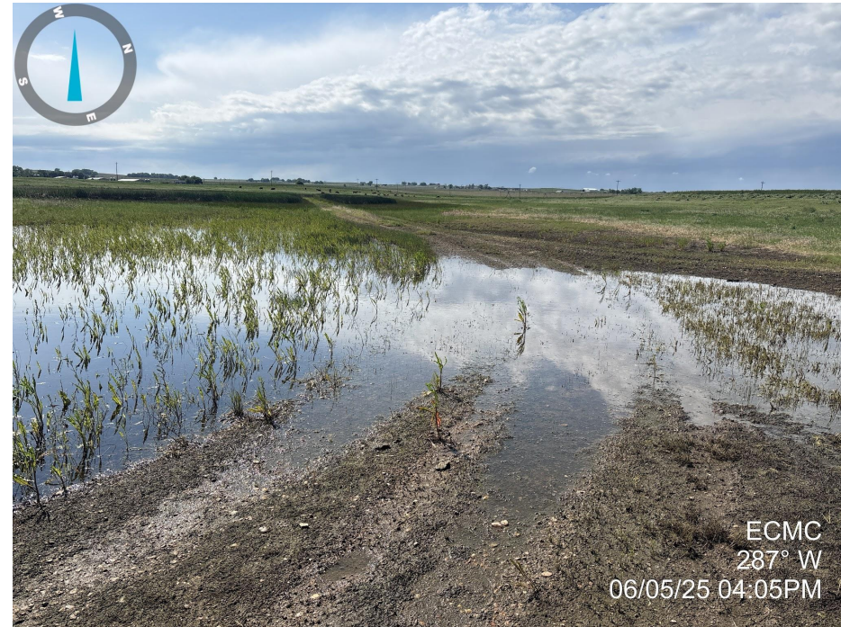
Photo 6. Photo taken of the access road to the well location, facing west. Photo illustrates that final reclamation activities have not taken place and gravel and bare ground remain along the road. Flooding is present across the access road from the adjacent wetland area.
