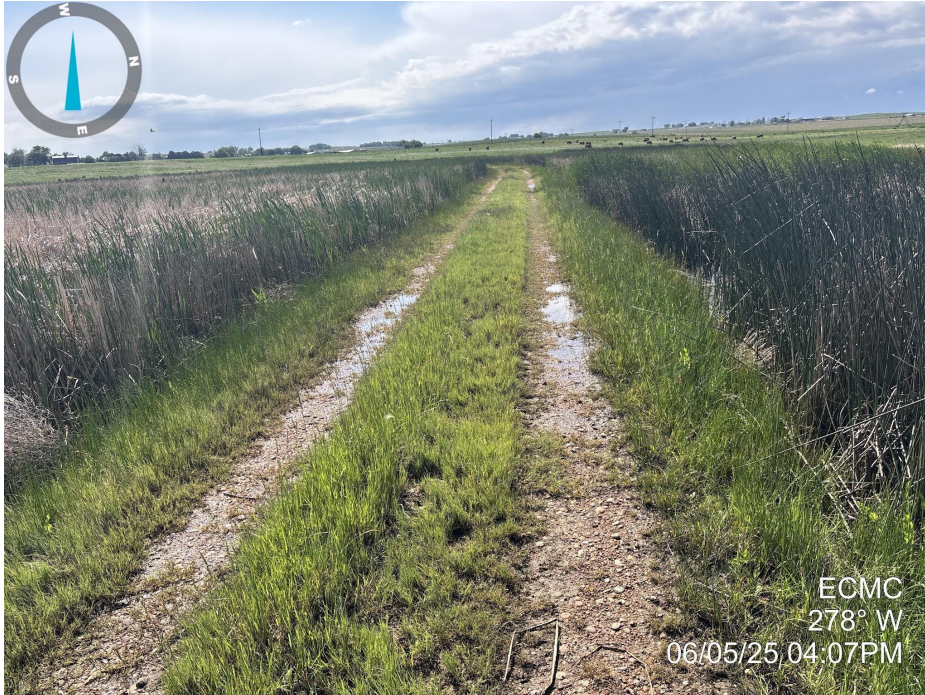
Photo 7. Photo taken of the access road to the well location, facing west towards the well location. Photo illustrates that final reclamation activities have not taken place and gravel and bare ground remain along the road.
