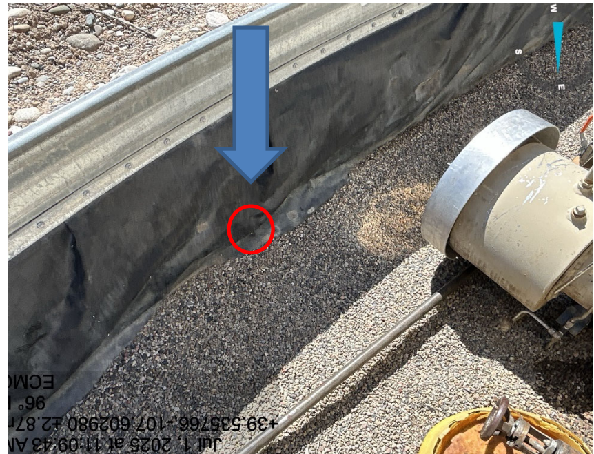
Hole in containment
