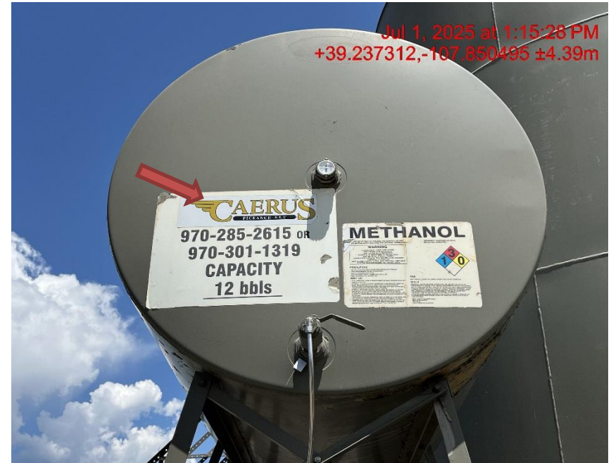
Photo # 9271 Label on methanol tank has incorrect operator name
