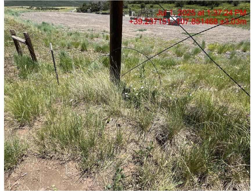
Photo # 9288 Loose barbed wire fencing/wildlife hazard
