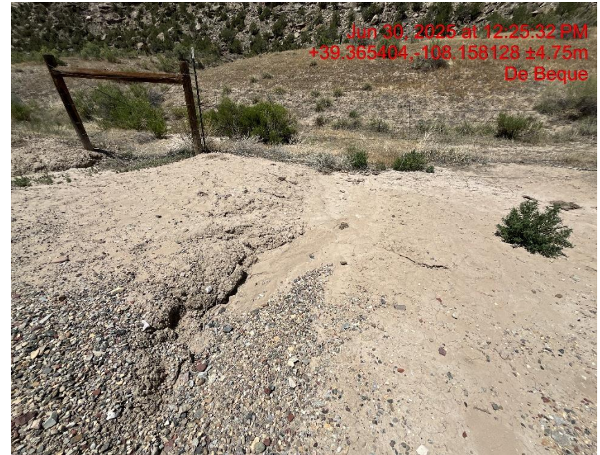
Photo # 9166 Failure to minimize erosion & transport of sediment/insufficient BMP's
