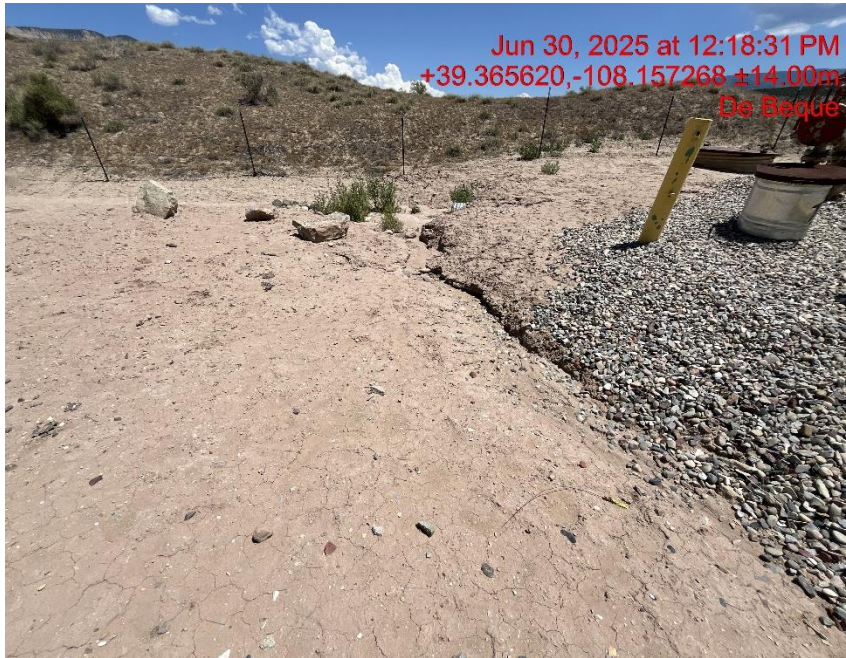
Photo # 9151 Failure to minimize erosion & transport of sediment/insufficient BMP's
