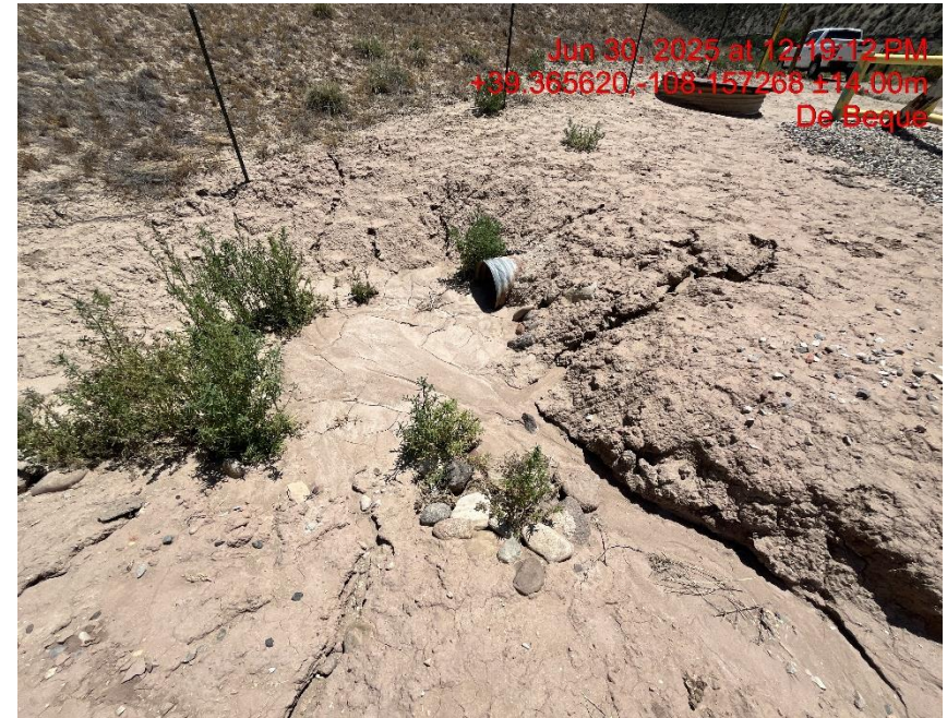
Photo # 9154 Failure to minimize erosion & transport of sediment/insufficient BMP's
