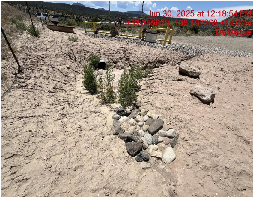
Photo # 9153 Failure to minimize erosion & transport of sediment/insufficient BMP's
