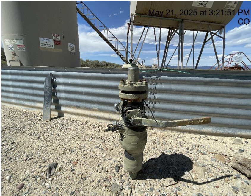
Photo # 2213 From inspection/audit 708906562 conducted on 05/21/2025 Unused flowline lacks lockout tagout (OOSLAT)
