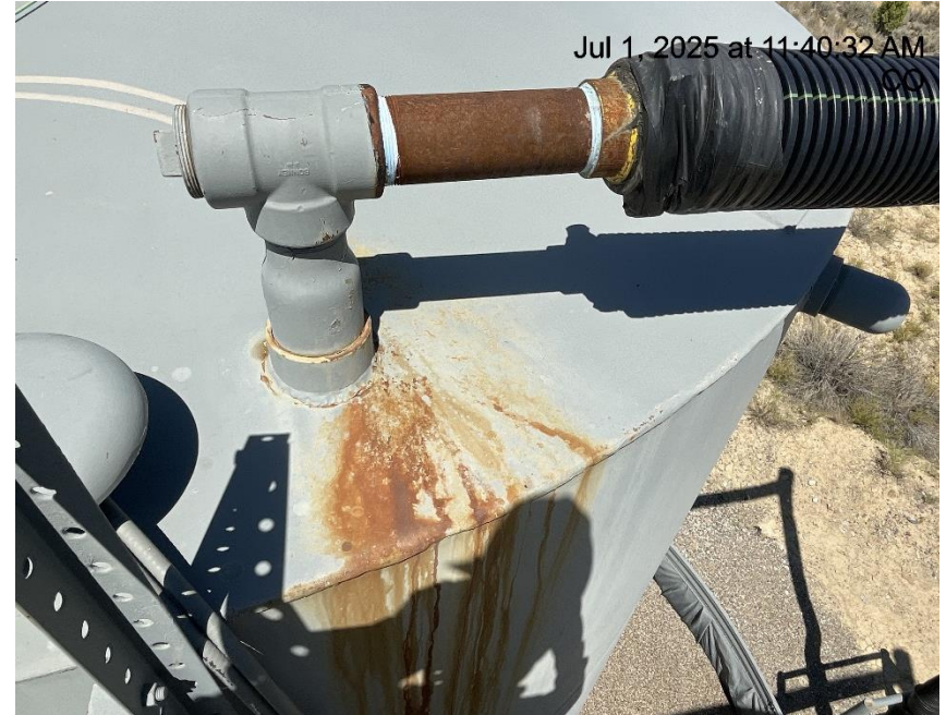
Photo # 9047 Possible tank failure
