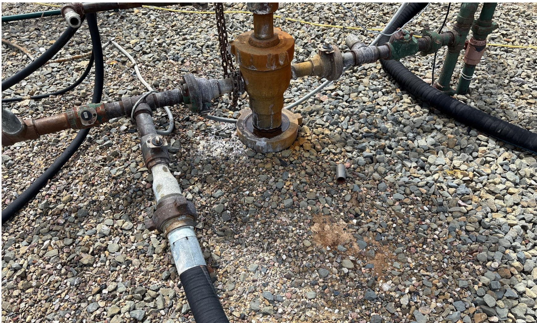
PHOTO 4: Bradenhead inaccessible. Install appropriate fittings to allow bradenhead visual inspection as per Rule 419.a.(1), (2). CA DATE 7-12-2025.
