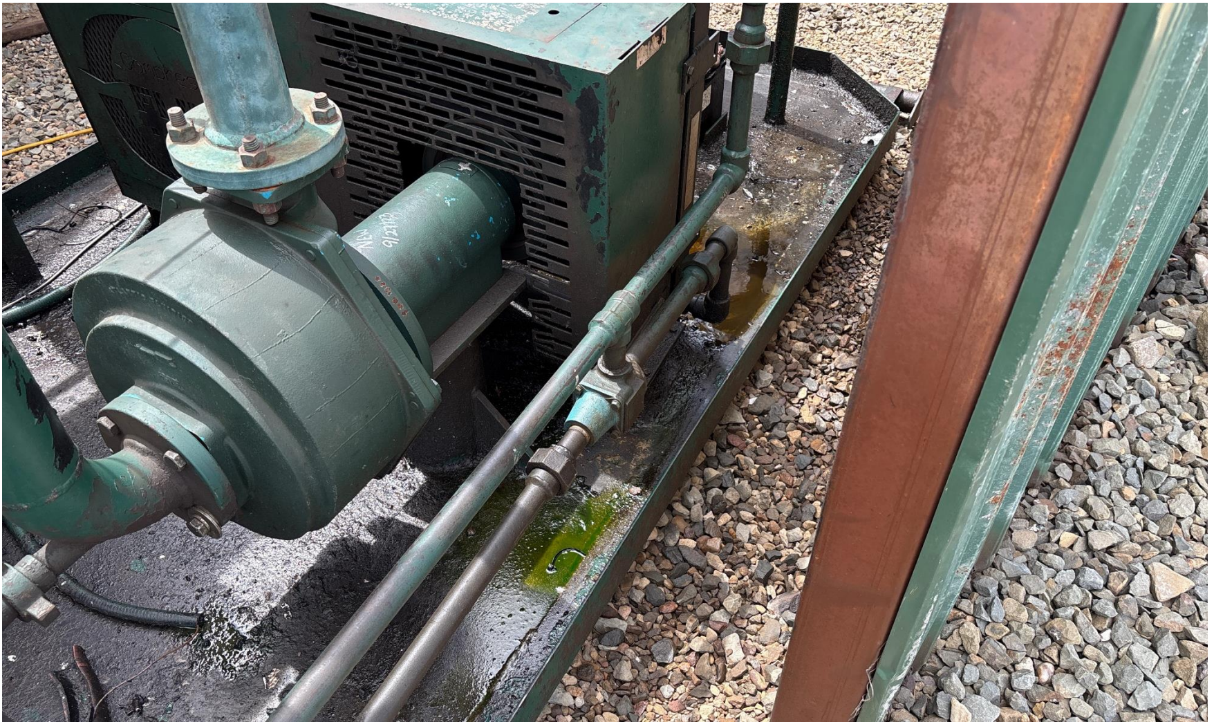
PHOTO 5: ANTIFREEZE AND OILY WASTE IN COMPRESSOR SKID. DRAIN OILY WASTE REPAIR ALL LEAKS AND REMOVE IMPACTED SOIL PER RULE 1002..(2).D & 1002.f.(2)B, Comply with general provisions of the oil and gas act for wildlife protection AND SB-181. CA DATE 7-2-2025.
