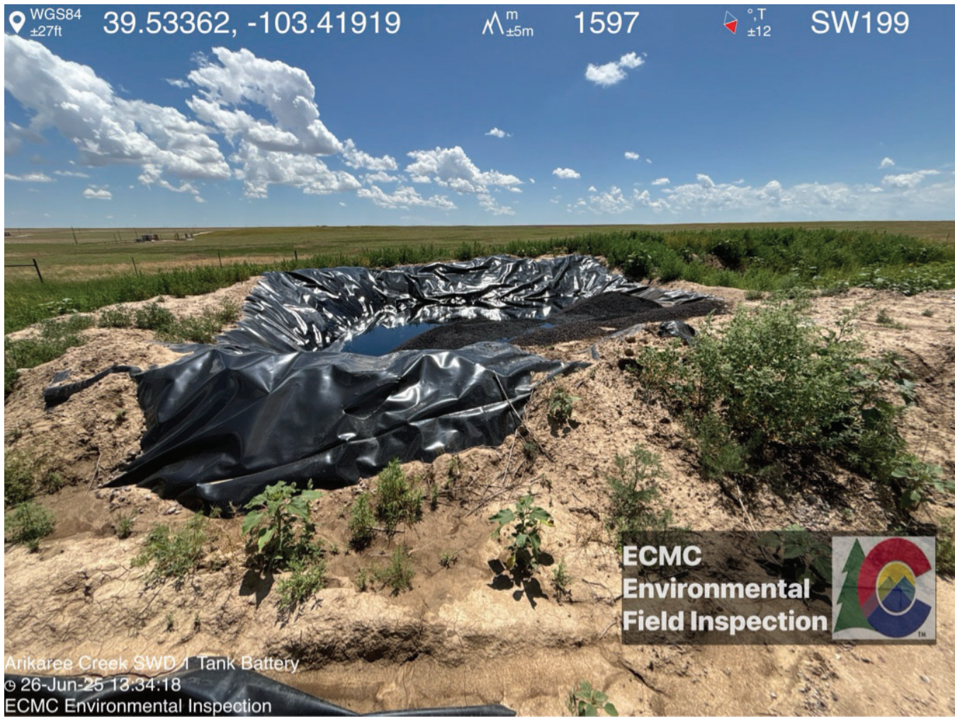
E&P waste stockpiled in bermed and lined containment Weeds
