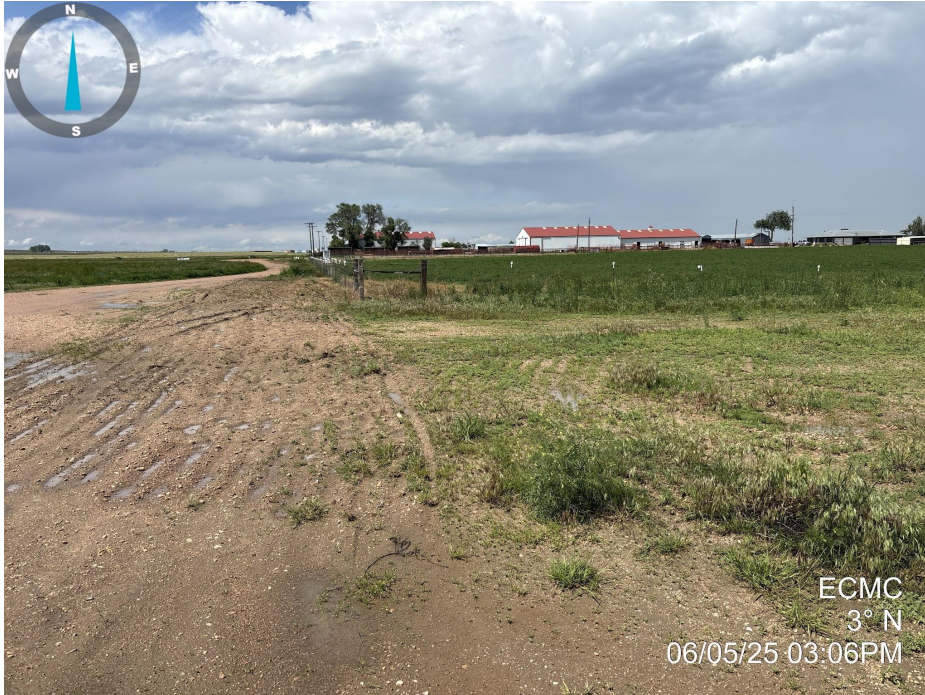
Photo 5. Photo taken the tank battery location, facing North. Photo illustrates that final reclamation activities have taken place, with evidence of drill row seeding, but vegetation establishment does not meet Rule 1004 standards.
