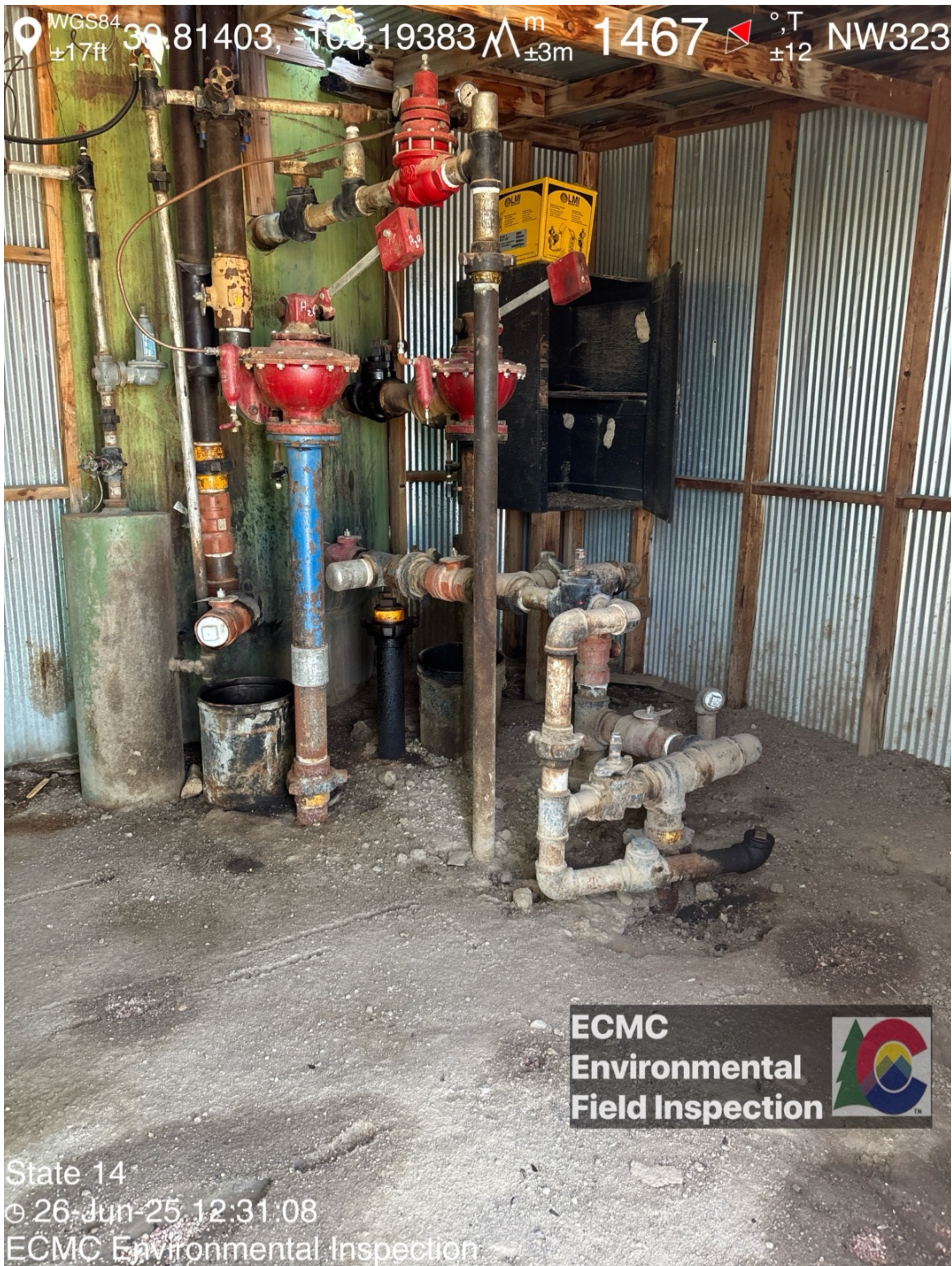
Stained soil observed within heater treater shed
