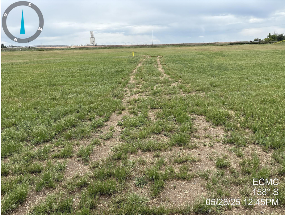
Photo 7. Photo taken of the access road, facing South towards the well location. Photo illustrates that vegetation establishment along the access road does not meet Rule 1004 standards and gravel remains across the location.
