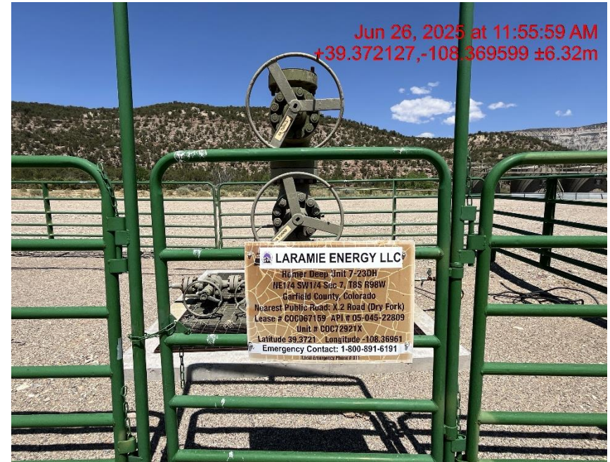
Photo # 8861 Wellhead sign is not legible/not in compliance with CECMC rules
