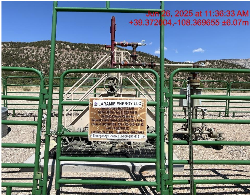
Photo # 8848 Wellhead sign is not legible/not in compliance with CECMC rules
