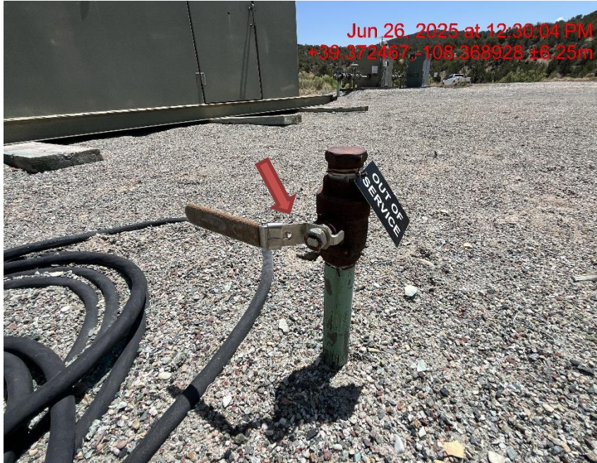
Photo # 8894 Unused flowline does not comply with CECMC 600 & 1100 series rules
