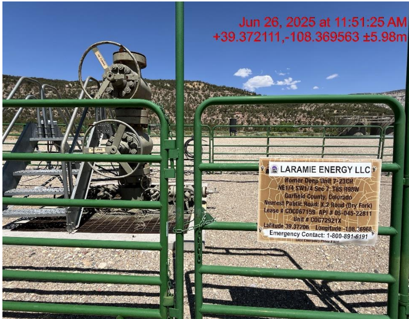
Photo # 8858 Wellhead sign is not legible/not in compliance with CECMC rules
