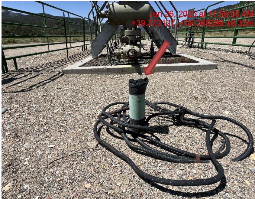
Photo # 8866 Unused flowline does not comply with CECMC 600 & 1100 series rules
