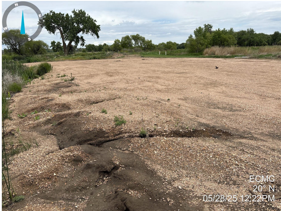
Photo 11. Photo taken of the access road, facing North towards the tank battery location. Photo illustrates stormwater erosion along the western portion of the access road.
