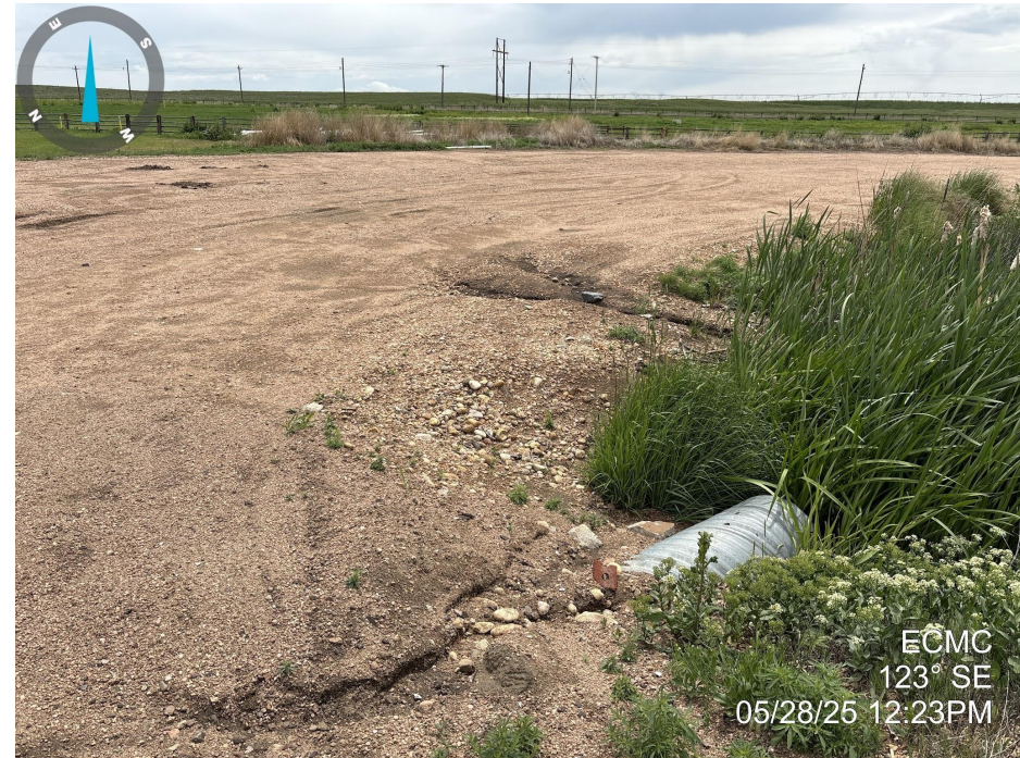
Photo 12. Photo taken of the access road adjacent to the tank battery location, facing Southeast. Photo illustrates erosion along the edge of the access road and around the culvert.
