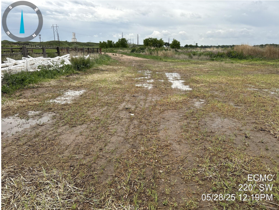
Photo 7. Photo taken of the access road, facing Southwest away from the location. Photo illustrates that final reclamation activities appear to have taken place, with evidence of drill row seeding and straw mulch, but vegetation has not established to Rule 1004 standards.
