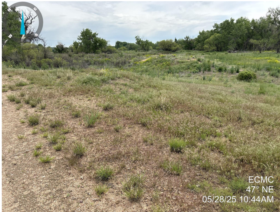
Photo 1. Photo taken of the northern portion of the tank battery location, facing Northeast. Photo illustrates that final reclamation activities appear to have taken place, but gravel remains and vegetation has not established to Rule 1004 standards. Weedy annual vegetation including cheatgrass ( Bromus tectorum ) was observed across the location.
