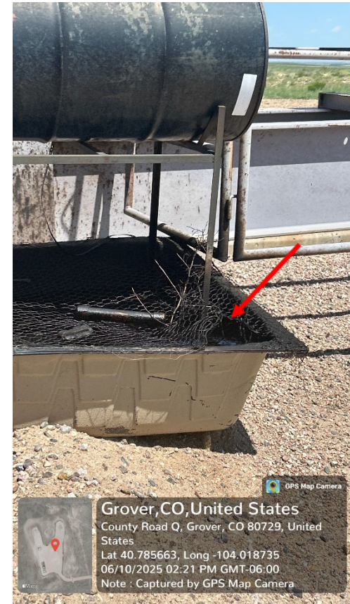
Photo 3 – Inadequate wildlife protection equipment
