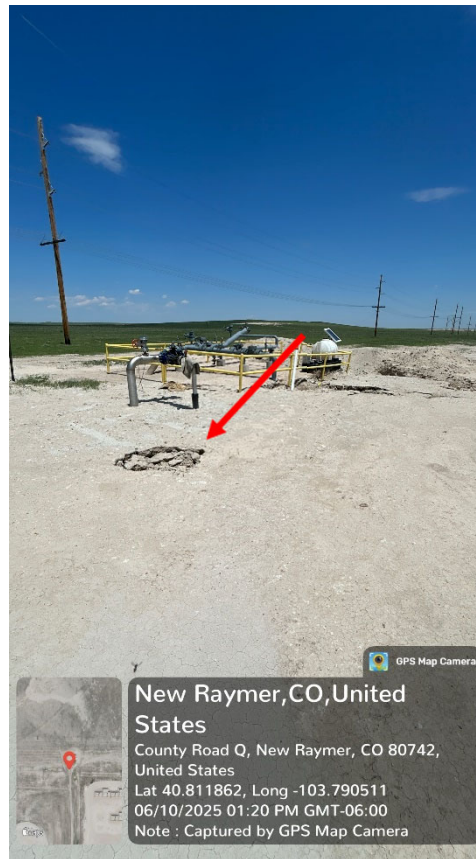
Photo 2 – Facing Northeast, collapsed backfill
