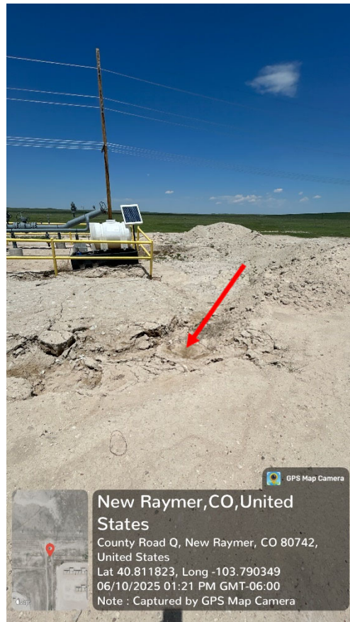
Photo 4 – Facing North, collapsed backfill
