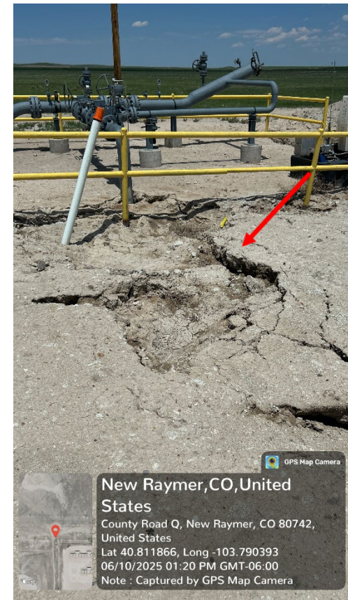
Photo 3 – Facing North, collapsed backfill
