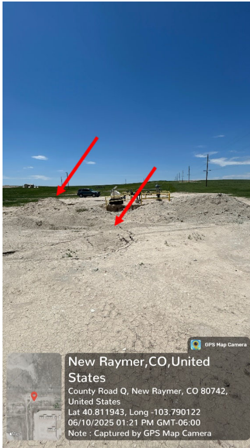
Photo 6 – Stockpile and collapsed backfill
