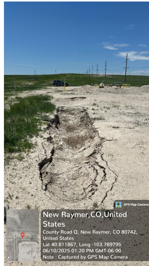
Photo 5 – Facing West collapsed backfill
