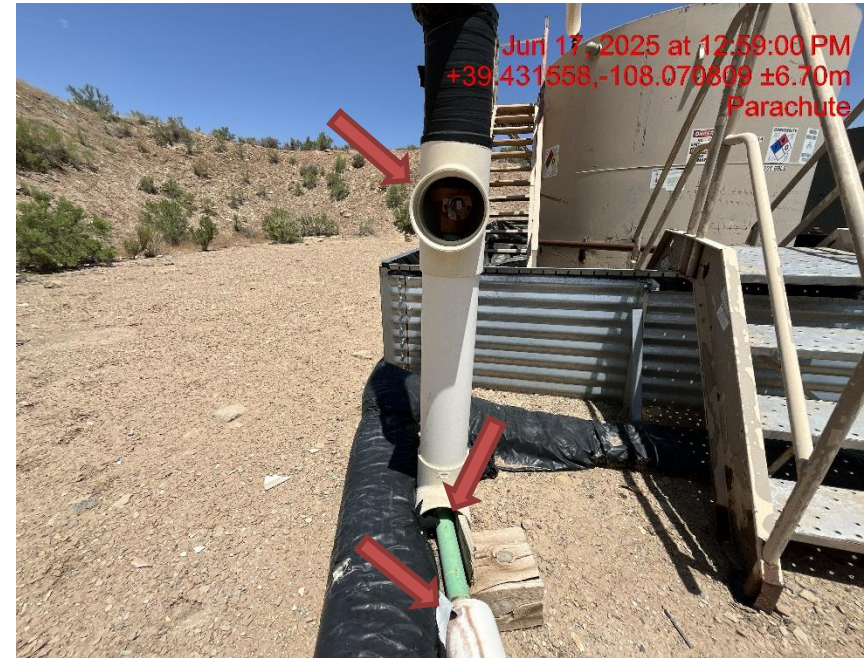
Photo # 8703 Flow line heating insulation open ended/wildlife hazard available for entry by wildlife
