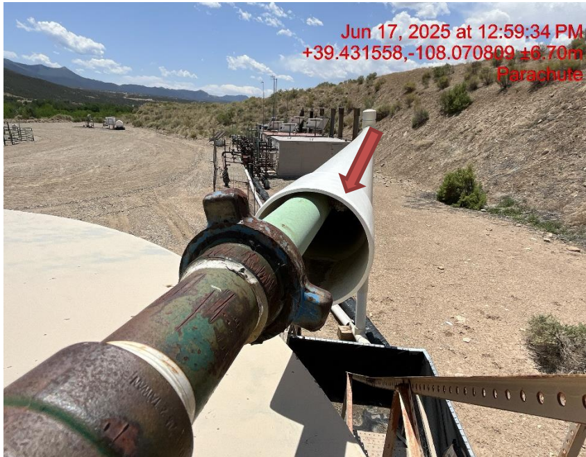
Photo # 8704 Flow line heating insulation open ended/wildlife hazard available for entry by wildlife
