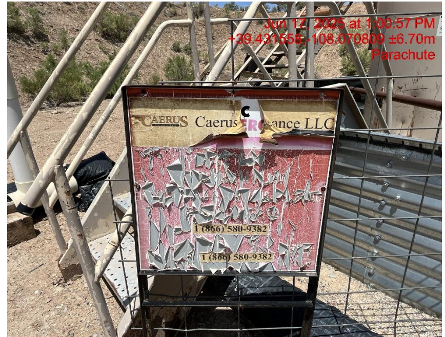
Photo # 8707 Battery signage is not legible/not in compliance with CECMC rules
