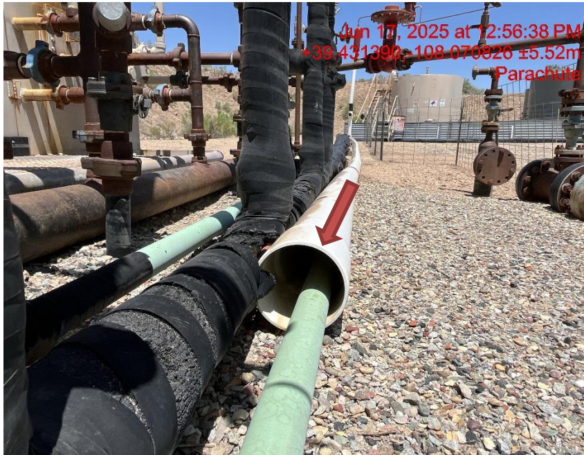
Photo # 8699 Flow line heating insulation open ended/wildlife hazard available for entry by wildlife
