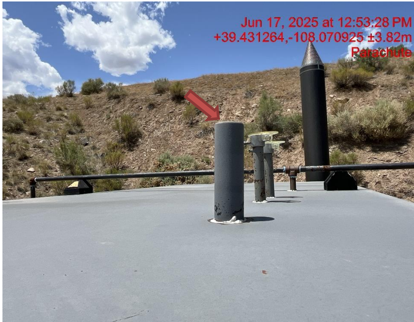
Photo # 8694 PRV vent line does not comply with CECMC pressure safety device rules
