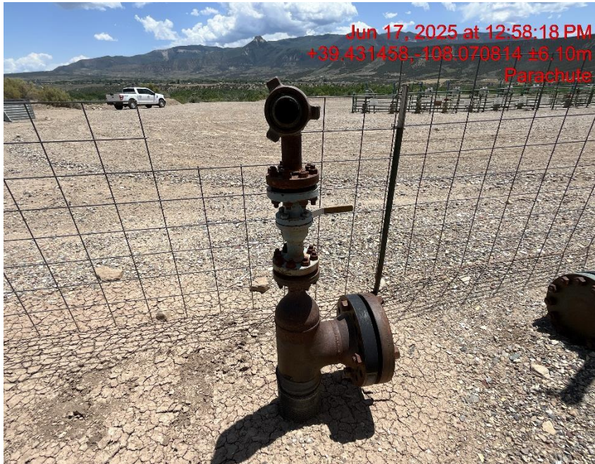
Photo # 8702 Unused flowline does not comply with CECMC 600 & 1100 series rules
