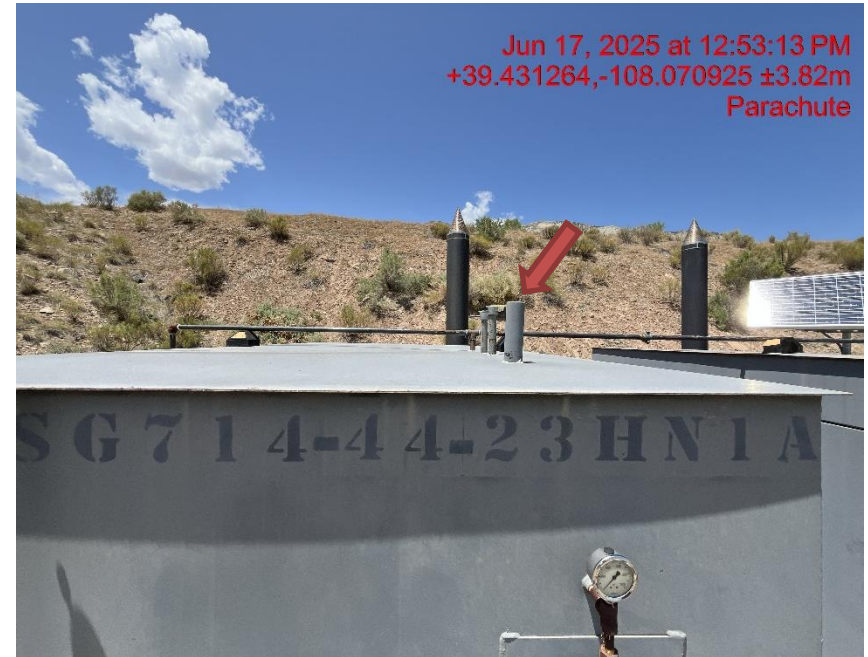
Photo # 8693 PRV vent line does not comply with CECMC pressure safety device rules
