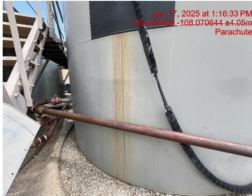
Photo # 8730 Suspected leaks on tank 1 production tank/tank appears to lack integrity
