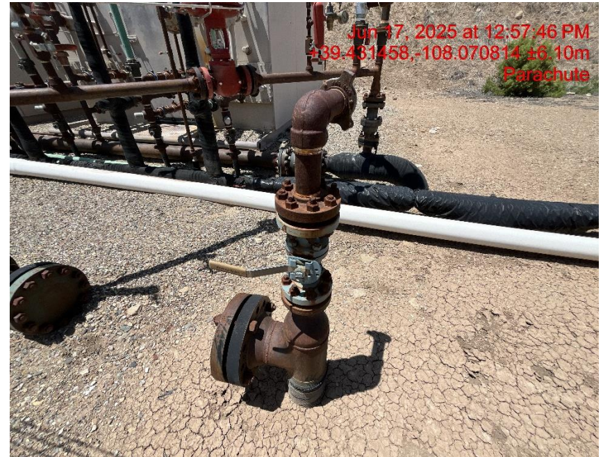
Photo # 8700 Unused flowline does not comply with CECMC 600 & 1100 series rules
