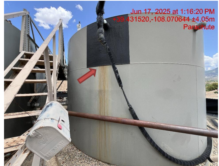
Photo # 8728 Suspected leaks on tank 1 production tank/tank appears to lack integrity
