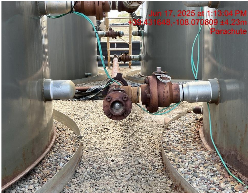
Photo # 8724 Open ended load line
