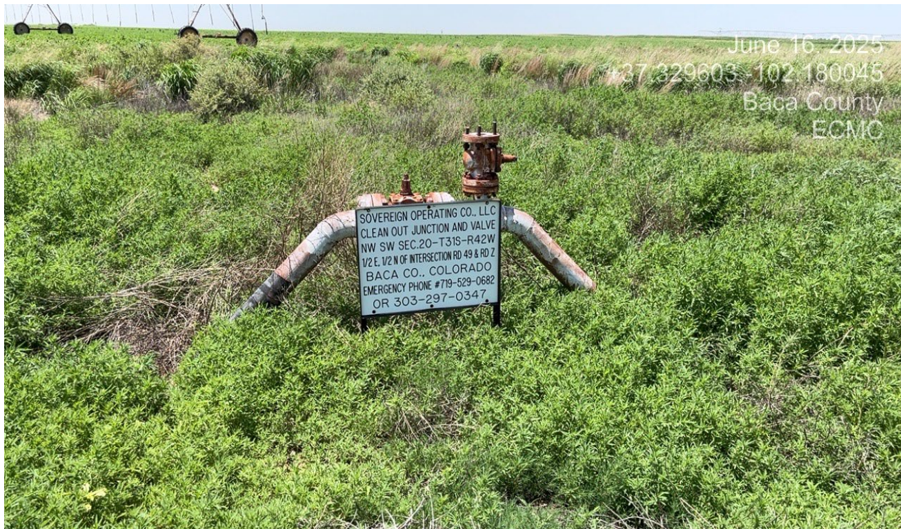
Photo 7. There was a cleanout junction 1850 ft. north of the pipeline previously observed. The cleanout junction is associated with the former gas compressor station and must be removed.
