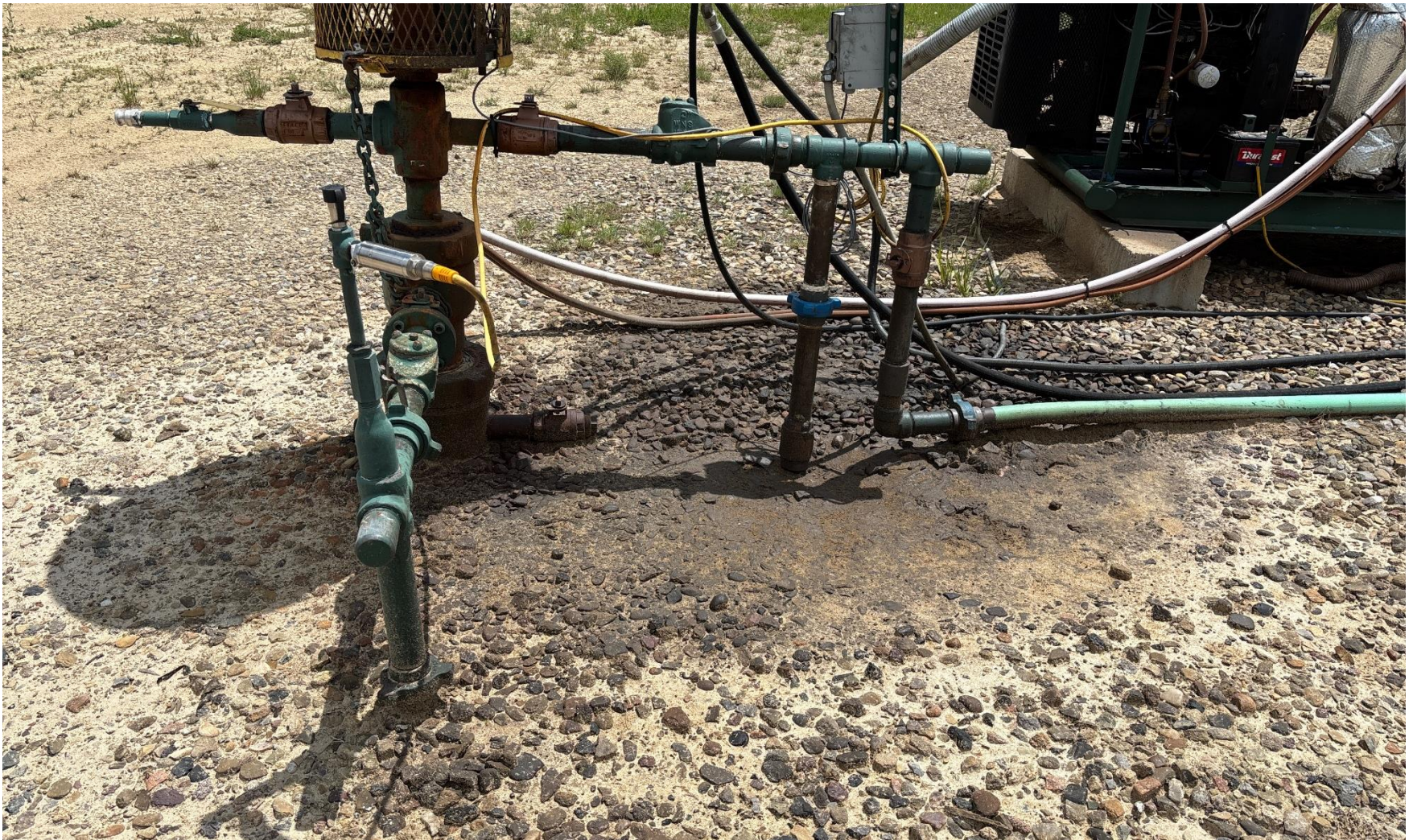
PHOTO 6: AREA OF IMPACTED SOIL NEAR TR WELLHEAD. Conduct maintenance on equipment, cleanup stained material and review self inspection processes. COMPLY WITH RULE 1002,. (2).D CA DATE 6-26-2025.
