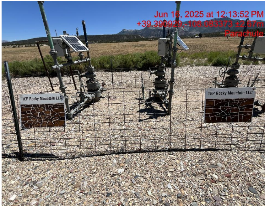
Photo # 8579 Wellhead signs are not legible
