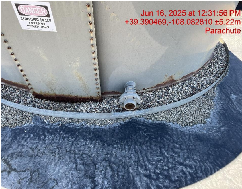
Photo # 8605 Open ended load line
