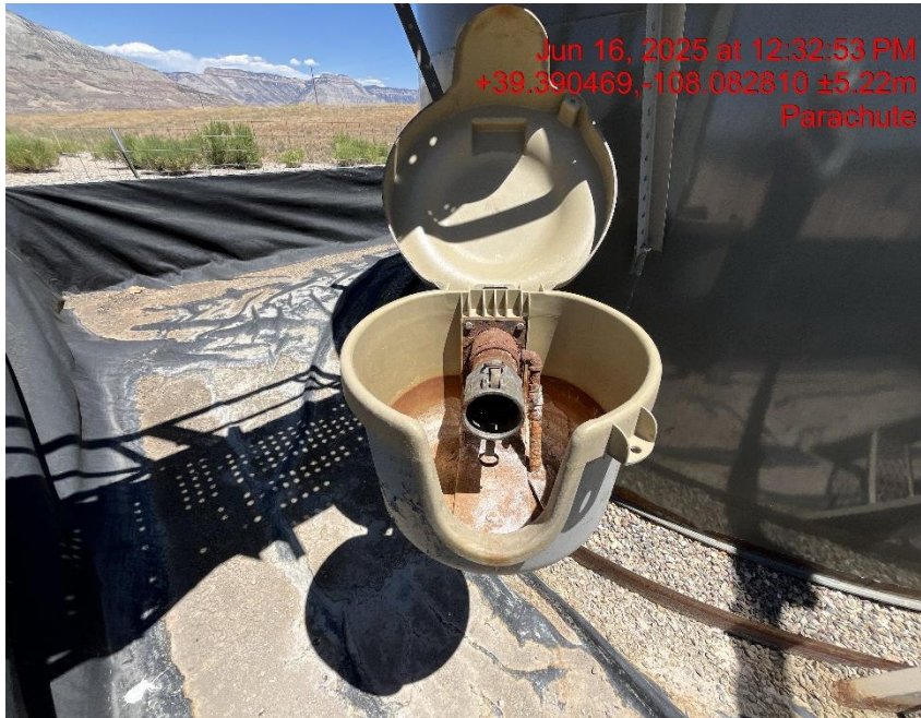
Photo # 8607 Open ended load line
