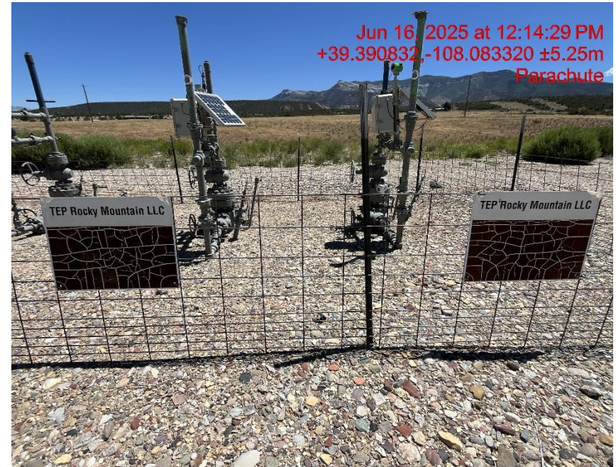
Photo # 8582 Wellhead signs are not legible
