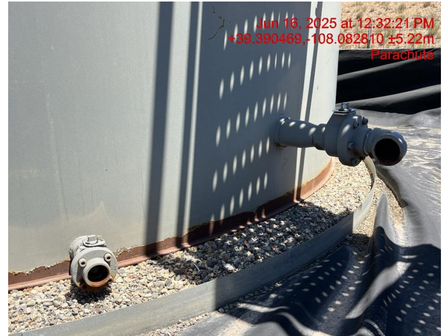
Photo # 8606 Open ended load lines
