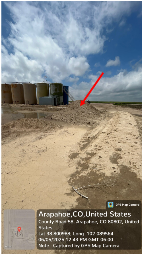
Photo 7 – Unlabeled stockpiles with inadequate berms
